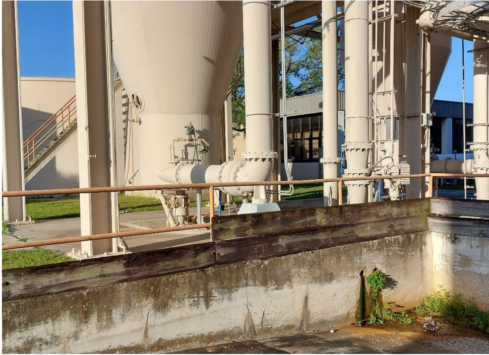
Photo 7 – LBP orange metal handrails around Structures 8a & 8b
