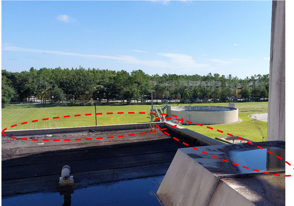
Photo 1 – ACM black asphalt roofing perimeter flashing on Structure 9
