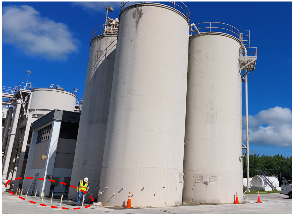
Photo 10 – LBP yellow on metal parking bollards of Structure 10
