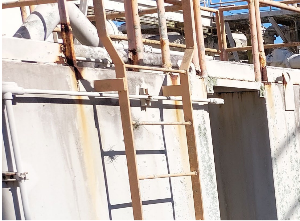
Photo 9 – LBP orange metal handrails on roof of Structure 9
