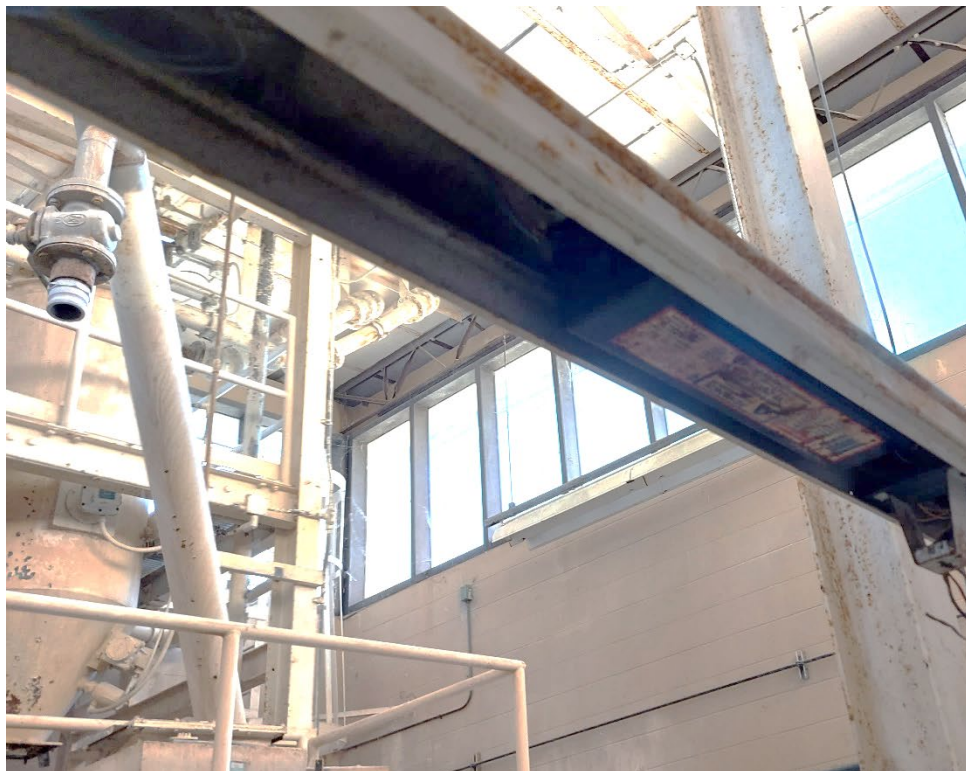
Photo 16 – Fluorescent light fixture with eight-foot bulbs (bulbs on ground)
