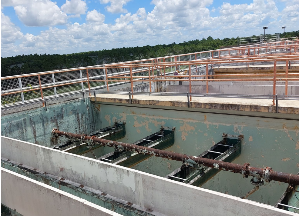
Photo 5 – LBP orange metal handrails on roof of Structure 6
