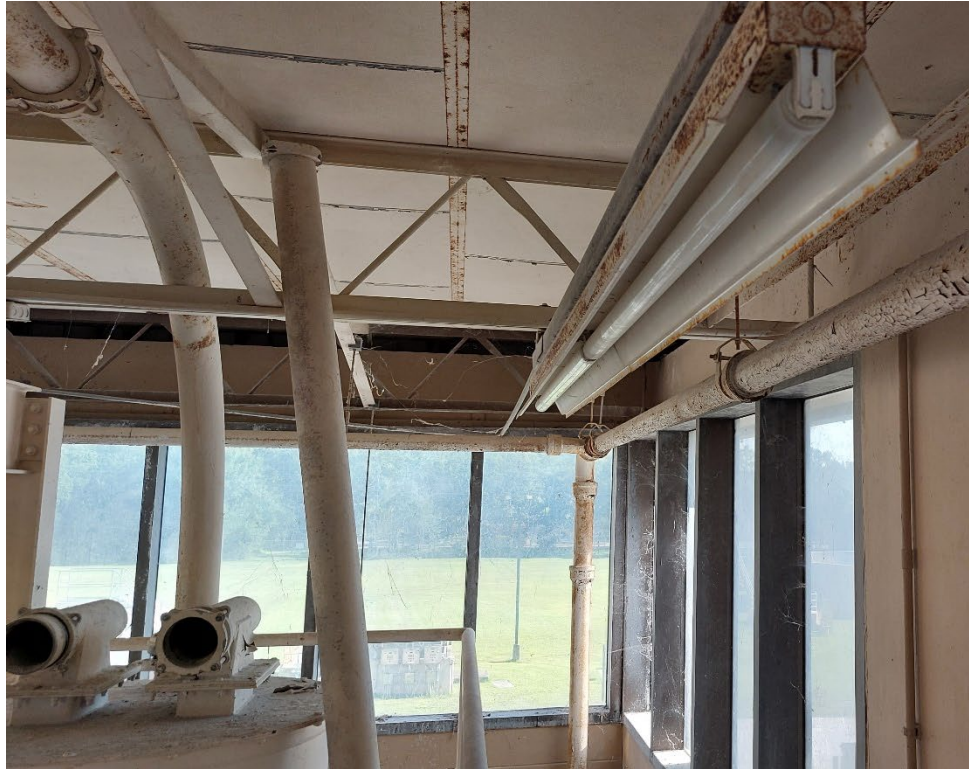
Photo 15 – Fluorescent light fixture with four-foot bulb
