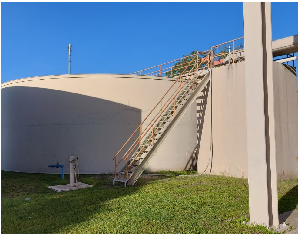
Photo 14 – LBP orange handrails on top of Structures 13 & 14
