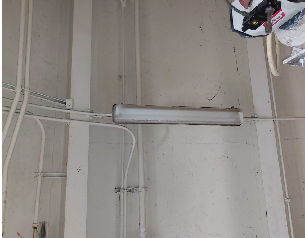
Photo 19 – Fluorescent light fixture with four-foot bulb
