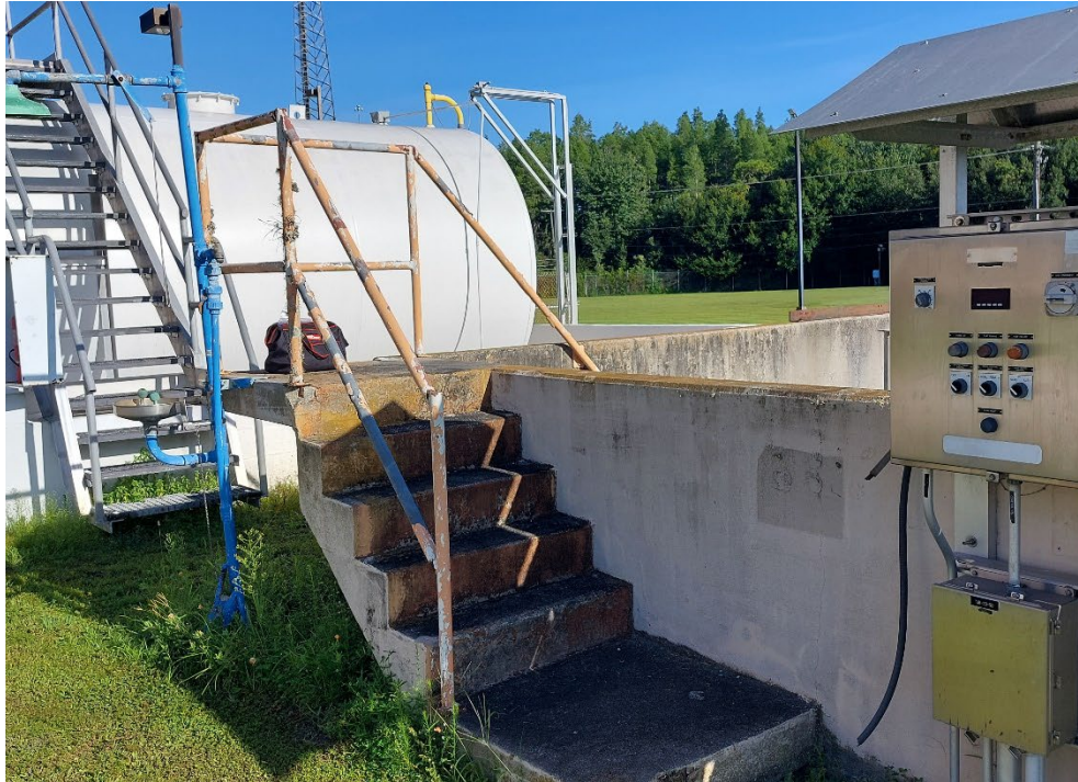
Photo 3 – LBP orange metal handrail on Structure 3
