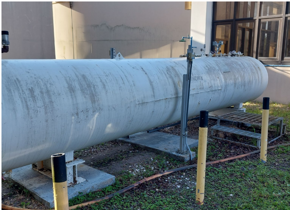
Photo 12 – LBP yellow metal parking bollards around Structure 11
