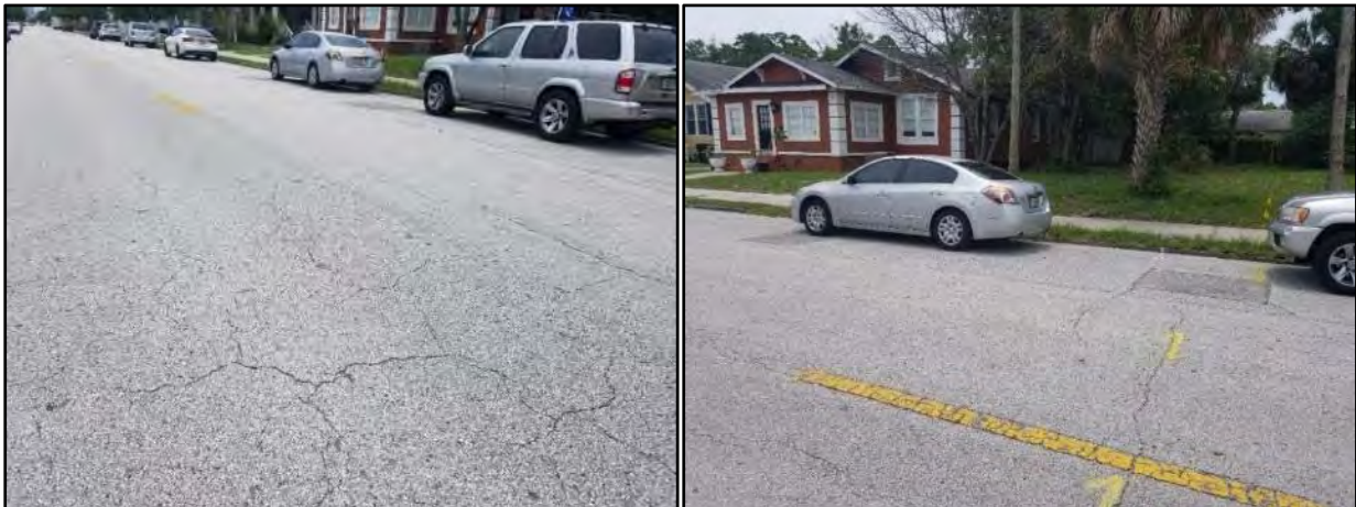
Figures 6 & 7: Block Cracking (300-ft. west of N. Fremont Avenue) Asphalt Patches / Transverse Cracking (270-ft. west of N. Fremont Avenue)
