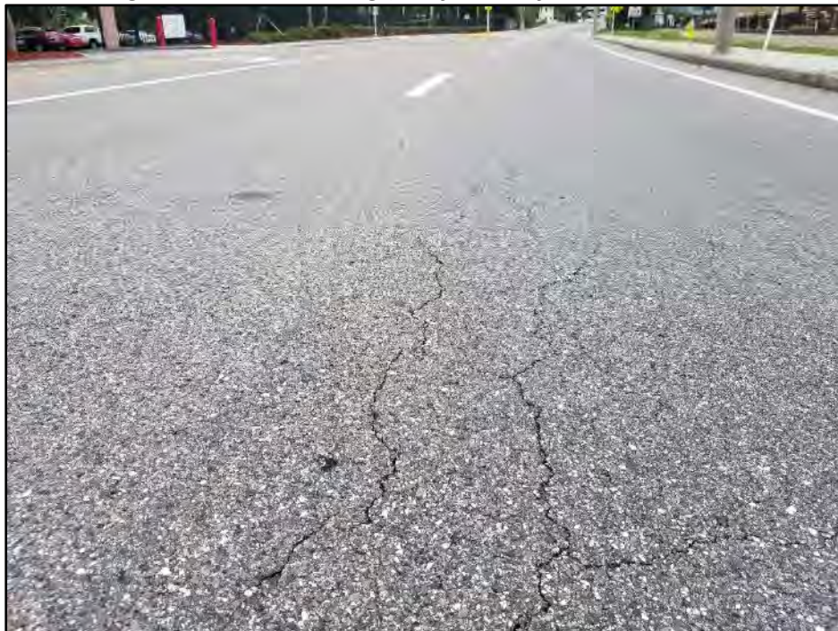
Figure 10: Block Cracking (335-ft. east of North Boulevard)
