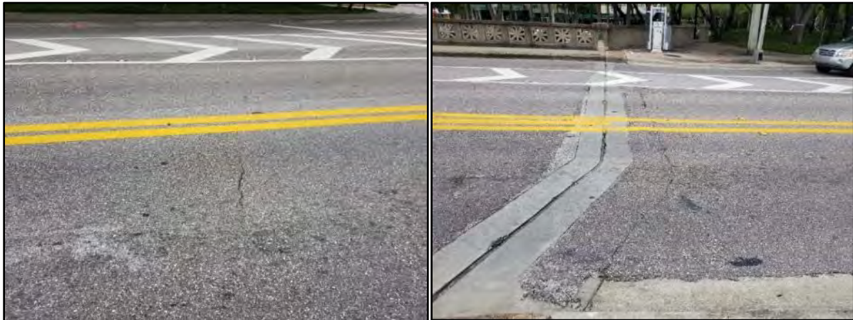
Figures 11 & 12: Transverse Cracking (200-ft. west of Doyle Carlton Drive) Reflection Cracking (240-ft. west of Doyle Carlton Drive)
