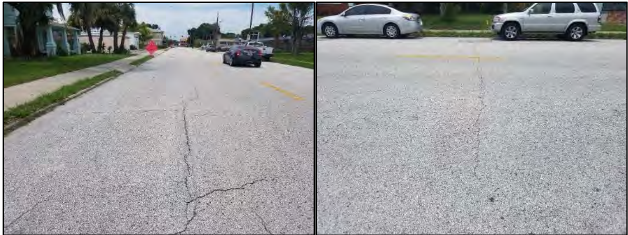
Figures 3 & 5: Longitudinal Cracking (250-ft. West of N. Fremont Avenue) Transverse Cracking (270-ft. west of N. Fremont Avenue)
