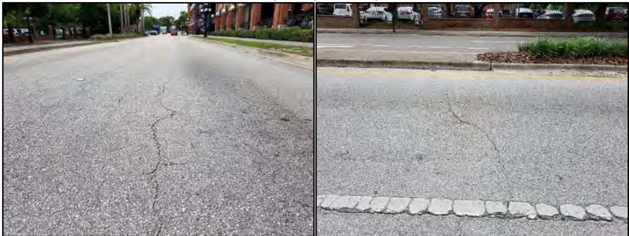
Figure 19 & 20: Longitudinal Cracking (40-ft. north of E. 8 th Avenue) Transverse Cracking (150-ft. north of E. 8 th Avenue)
