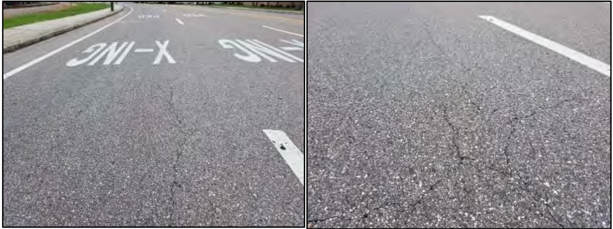
Figures 8 & 9: Longitudinal Cracking (330-ft. east of North Boulevard) Transverse Cracking (280-ft. east of North Boulevard)
