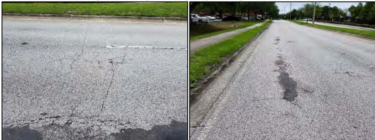
Figure 23 & 24: Transverse Cracking / Fatigue (Alligator) Cracking (70-ft. west of N. 14 th Street) Alligator Cracking / Patching (70-ft. west of N. 14 th Street)
