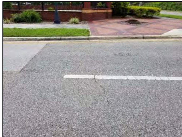
Figure 26: Transverse Cracking (45-ft. south of E. 13 th Avenue)
