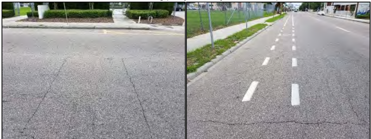
Figure 28 & 29: Transverse Cracking (160-ft. north of E. 17 th Avenue) Transverse Cracking (200-ft. north of E. 17 th Avenue)
