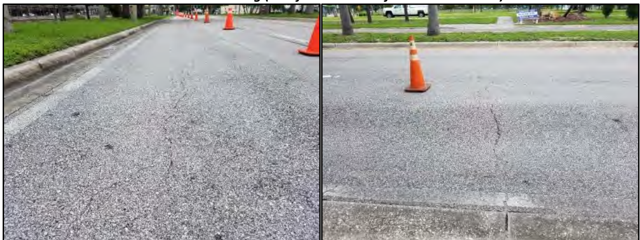
Figure 13 & 14: Longitudinal Cracking (400-ft. northeast of N. Nebraska Ave.) Transverse Cracking (430-ft. northeast of N. Nebraska Ave.)
