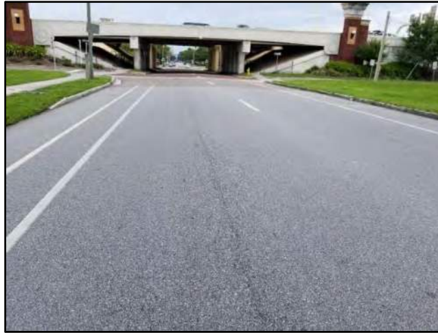
Figure 27: Transverse Cracking (125-ft. north of E. 14 th Avenue)
