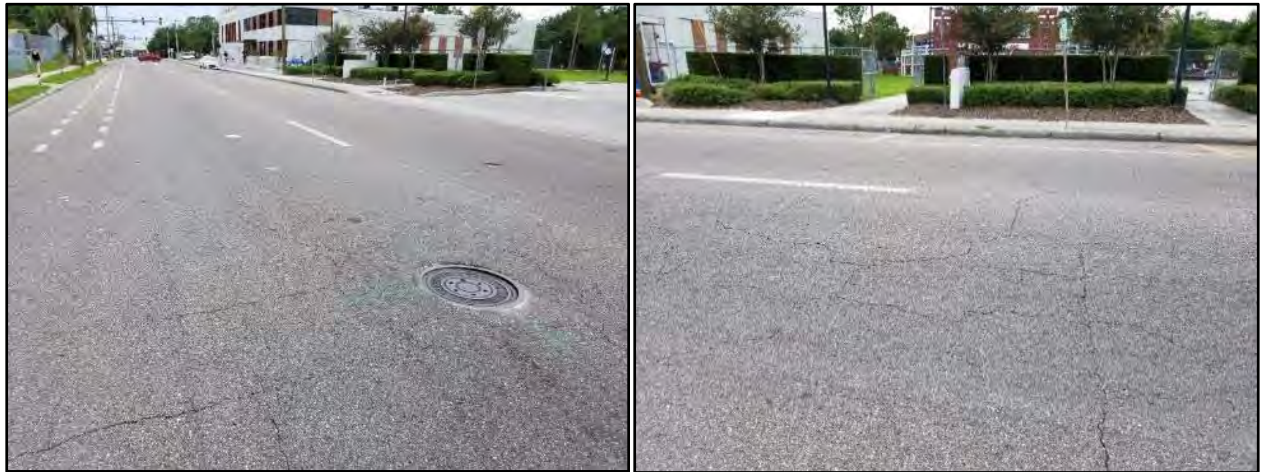
Figure 30 & 31: Longitudinal Cracking / Transverse Cracking / Block Cracking (240-ft. north of E. 17th Avenue) Block Cracking (150-ft. north of E. 17th Avenue)
