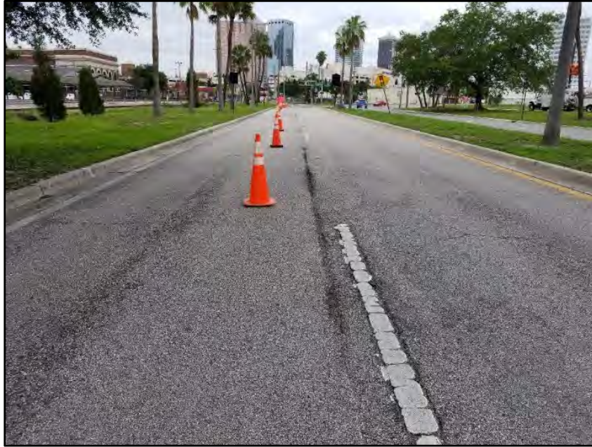
Figure 15: Transverse Cracking and Raveling (370-ft. northeast of N. Nebraska Ave.)
