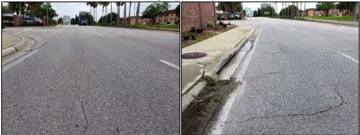
Figure 16 & 17: Longitudinal Cracking (30-ft. north of E. 6th Avenue) Transverse Cracking (80-ft. north of E. 6th Avenue)
