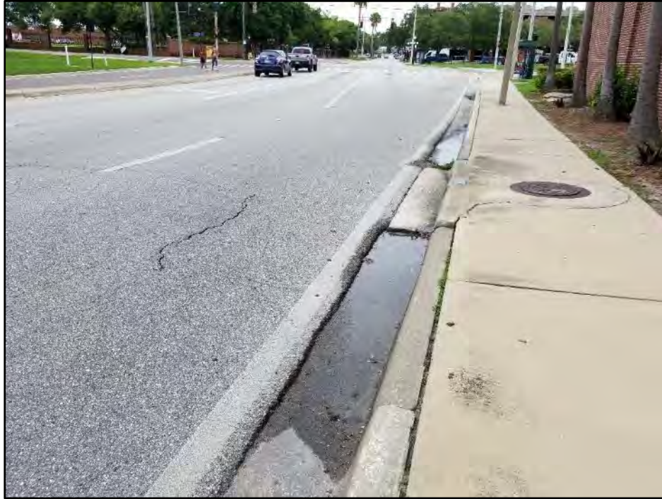
Figure 18: Poor Drainage (20-ft. north of E. 6th Avenue)
