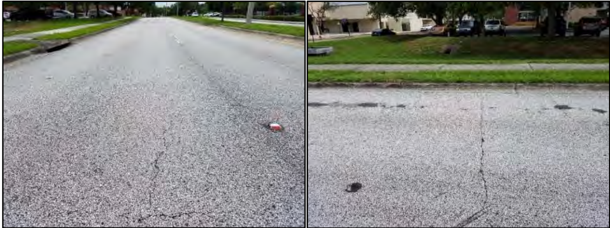
Figure 21 & 22: Longitudinal Cracking (150-ft. west of N. 14 th Street) Transverse Cracking (80-ft. west of N. 14 th Street)
