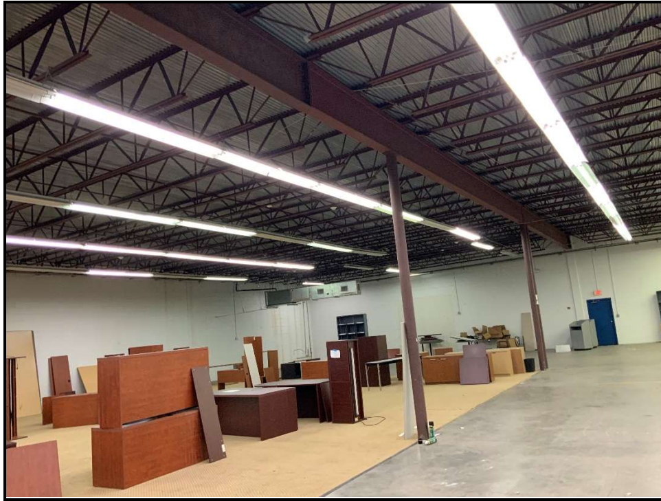
Photo 5: Steel frames placement. 6"Ø steel tube columns and W24 roof beams
