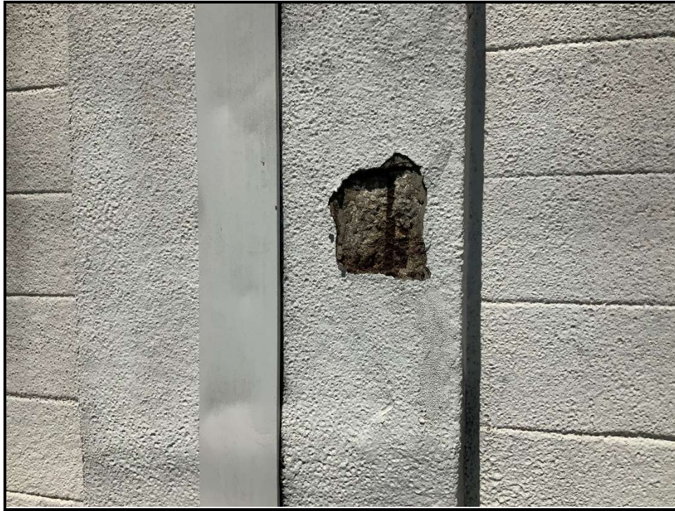
Photo 13: Concrete column spalling
