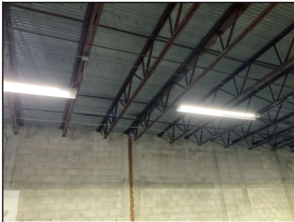
Photo 4: South west wing typical roof framing and construction/expansion joint
