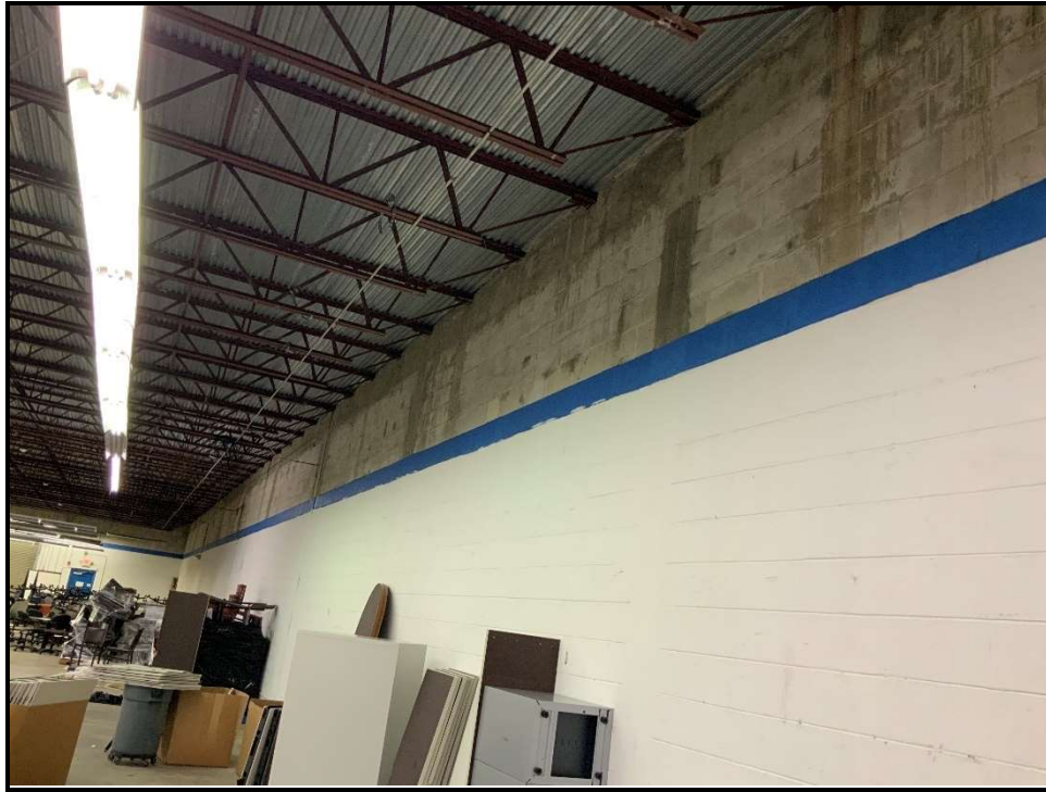
Photo 7: Typical interior bearing wall arrangement
