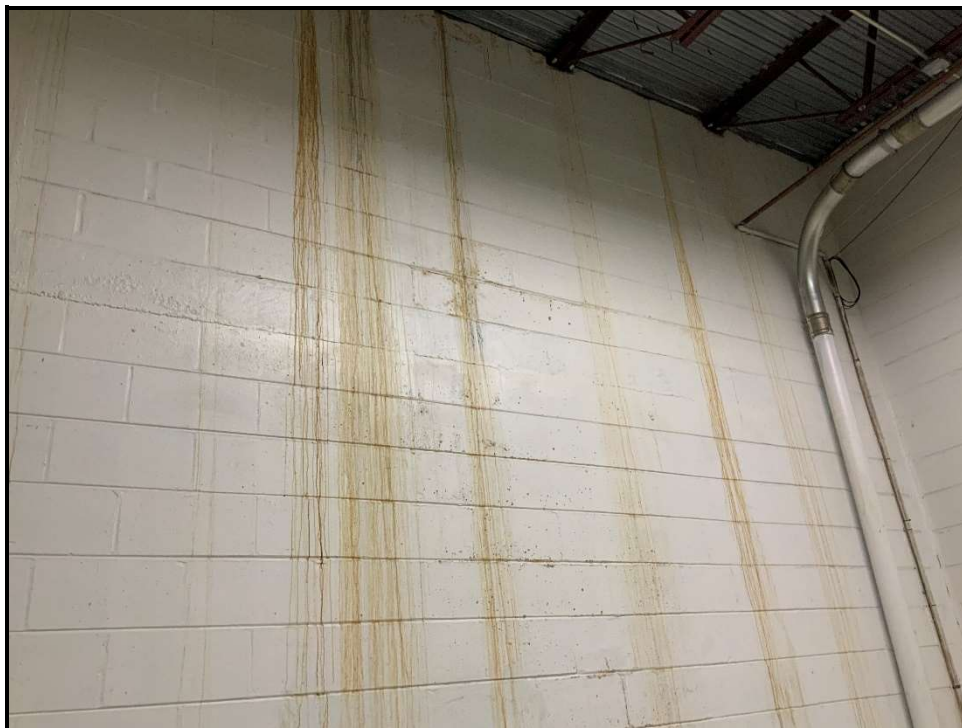
Photo 14: Sign of licking and rust
