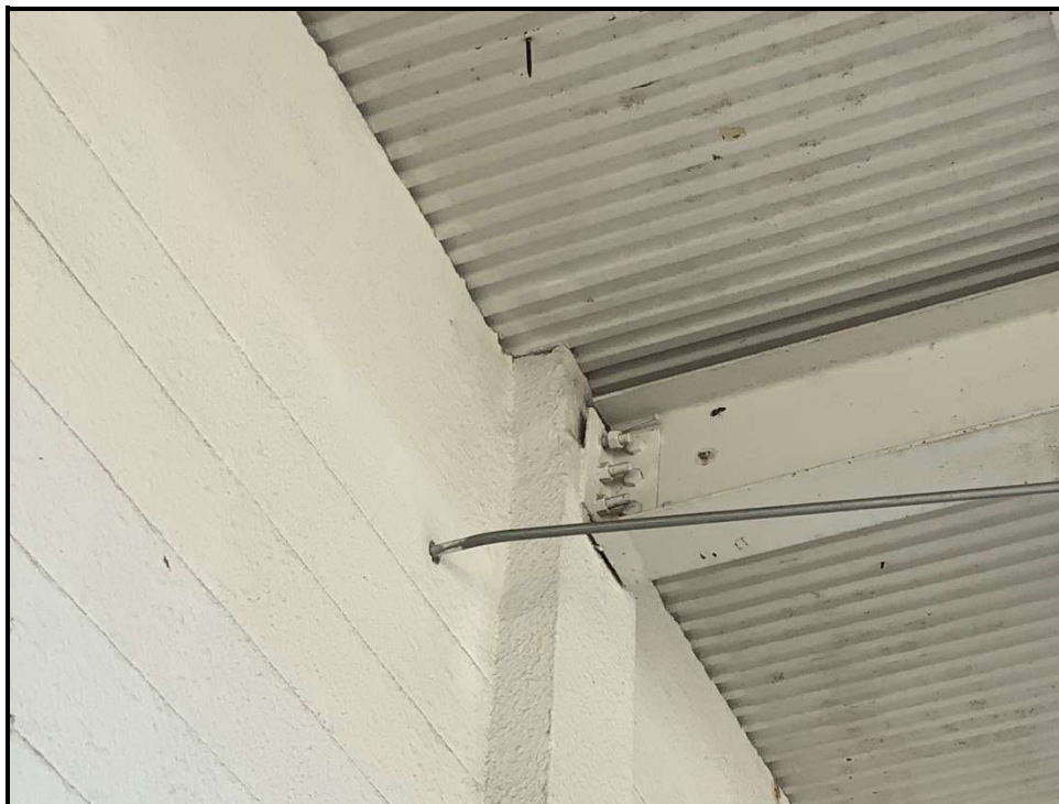
Photo 14: Loos bolt at frame connection
