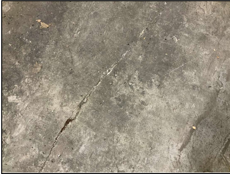
Photo 13: Typical slab on grade cracks
