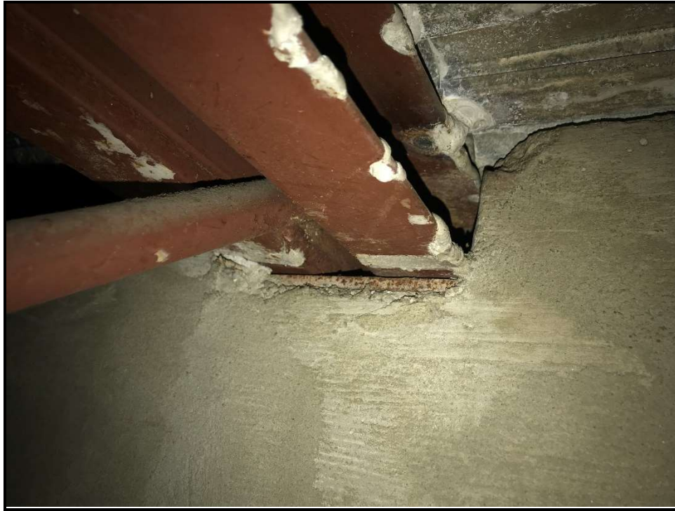
Photo 9: Typical roof joist seat at concrete tie beam.
