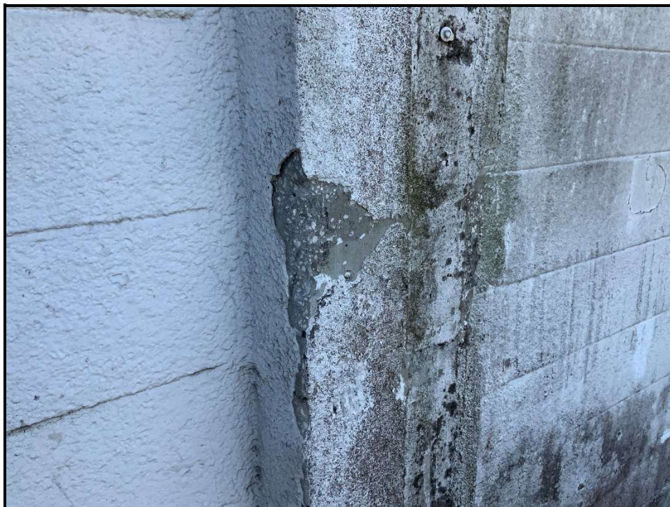
Photo 14: Concrete column spalling
