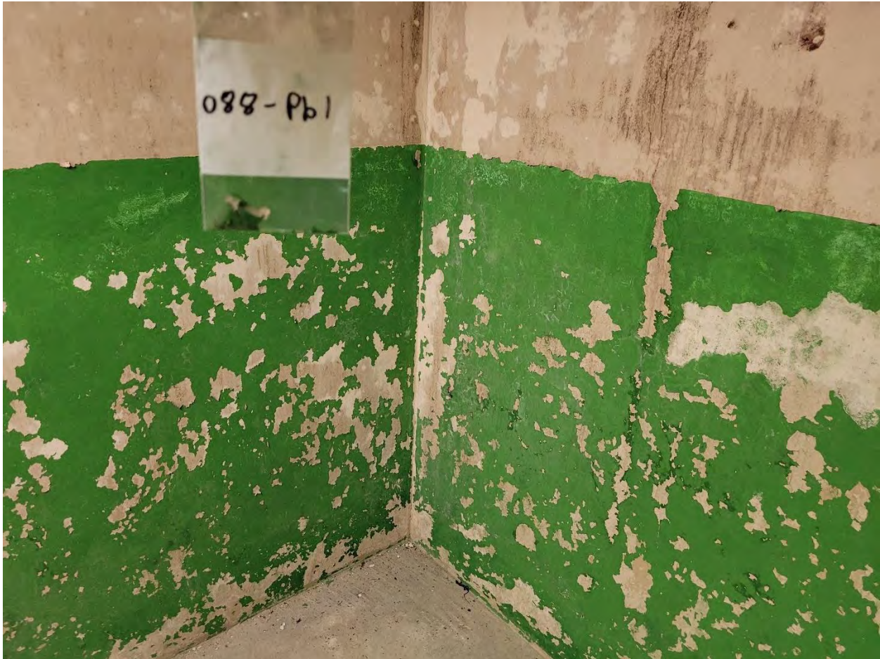
088-PB 1: Beige w/ Green Paint on Concrete Wall [NLD]
