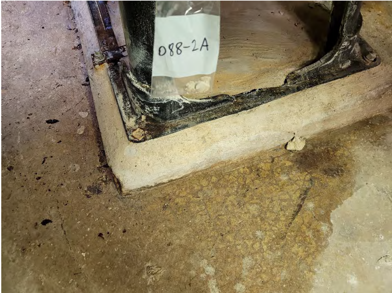
088-2A: Concrete Pedestals [NAD]
