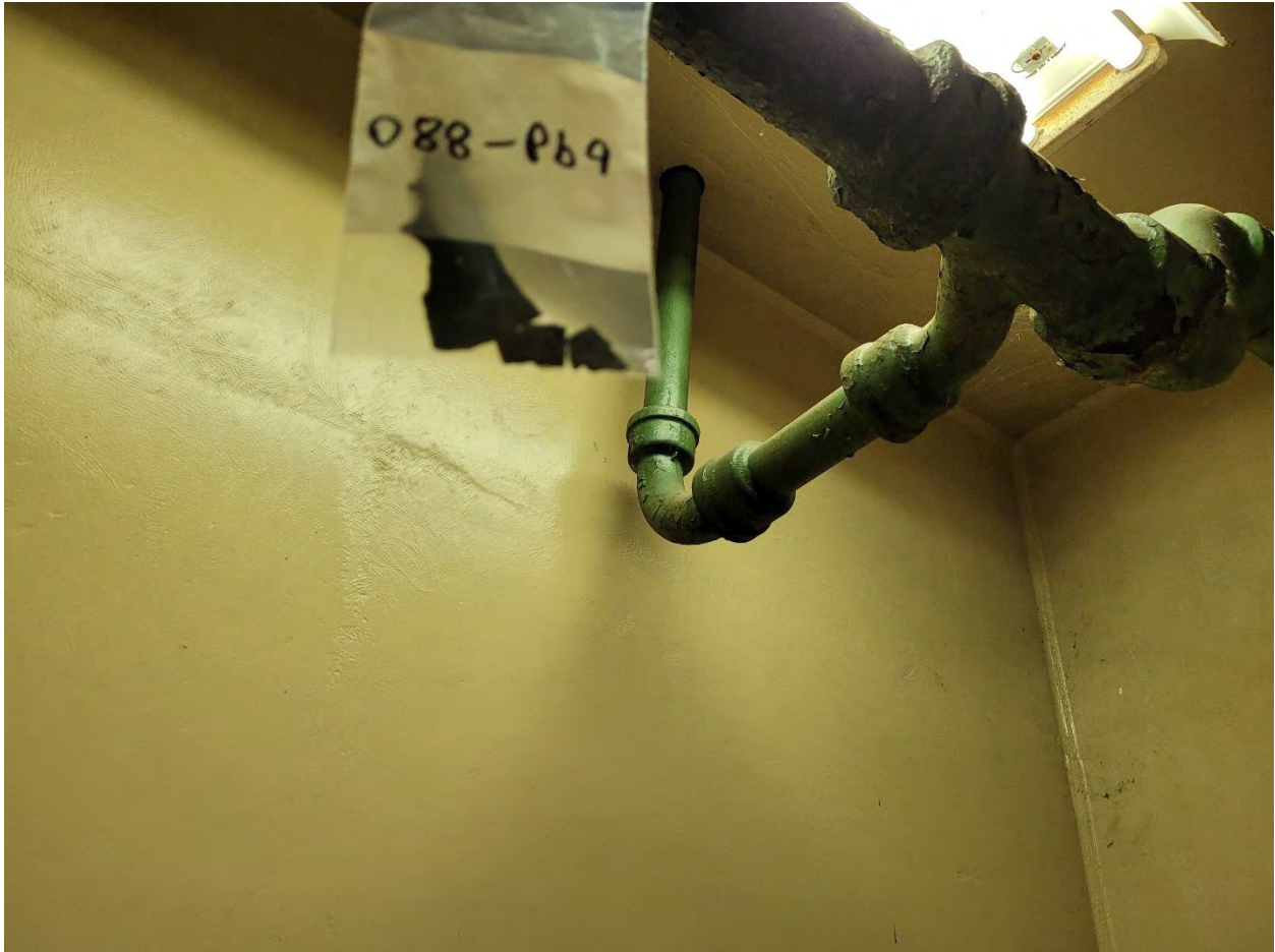
088-PB 9: Green Paint on Metal Pipe [0.024 % wt]
