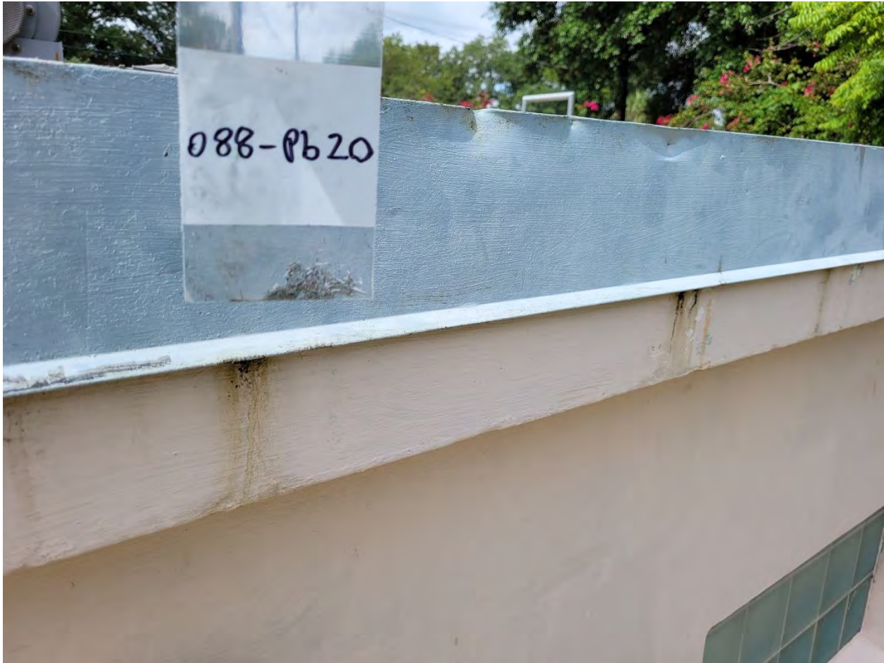
088-PB 20: Grey Paint on Metal [0.014 % wt]
