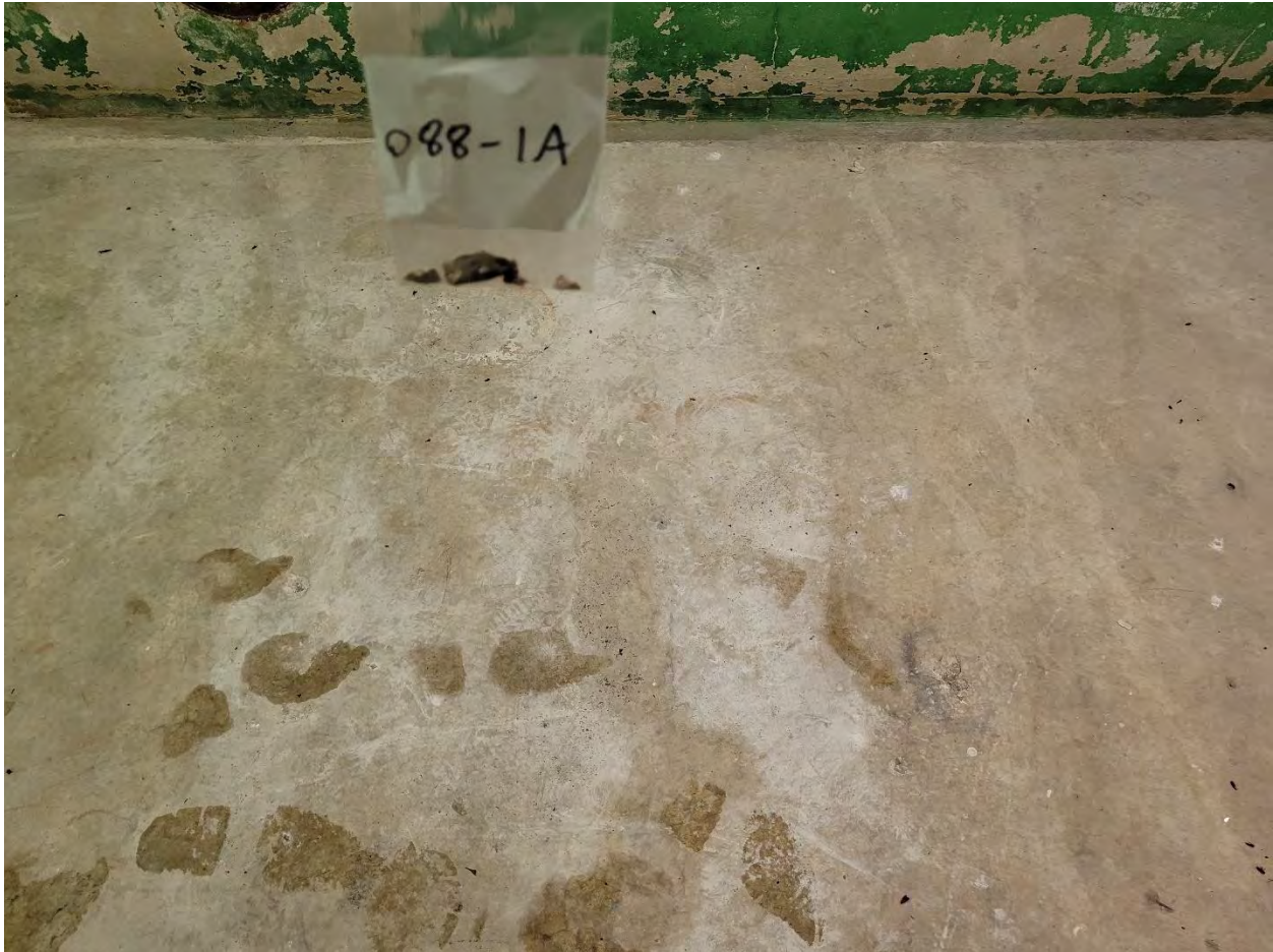
088-1A: Concrete Flooring/Walls [NAD]
