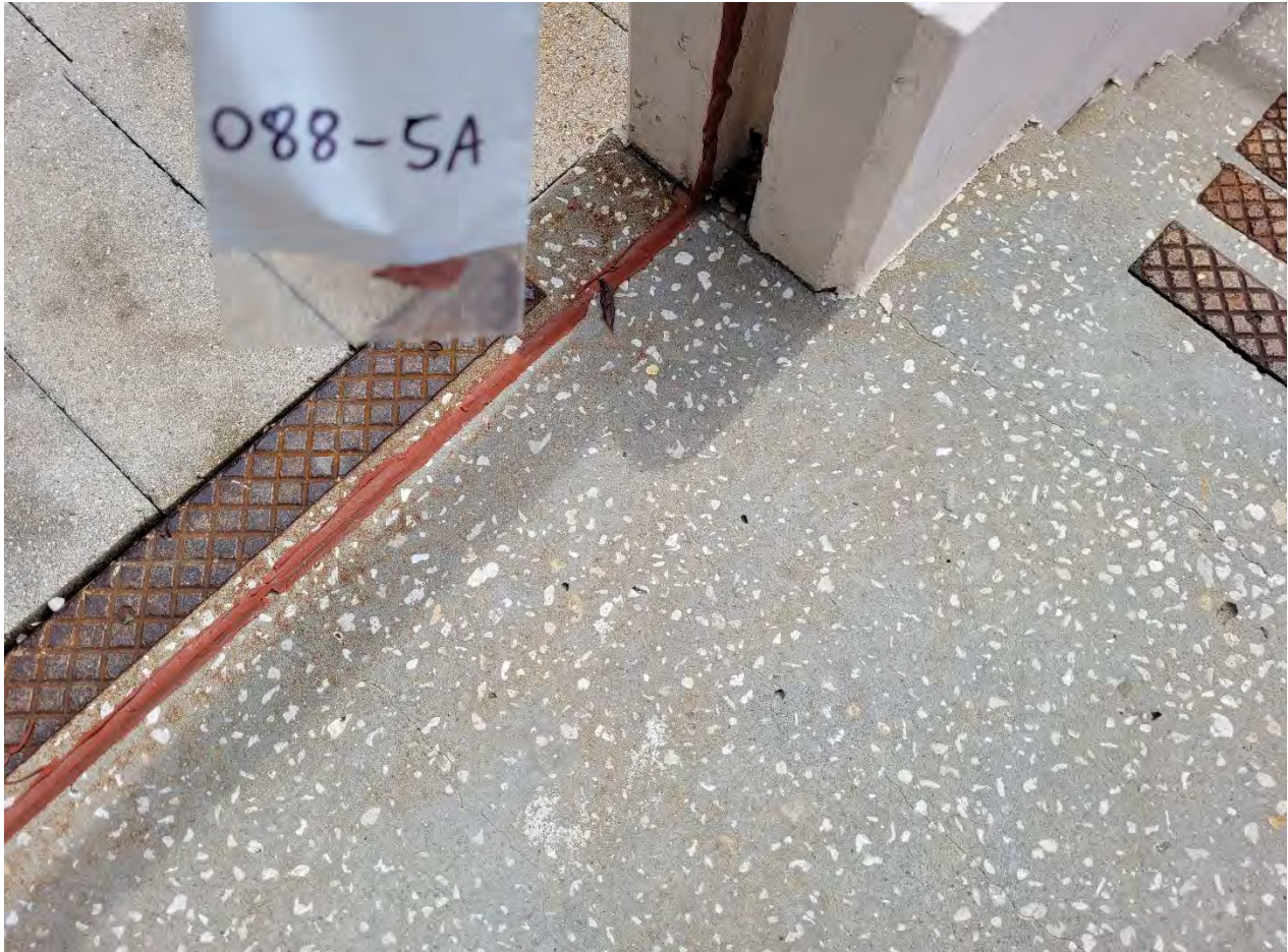
088-5A: Fire Caulking [NAD]
