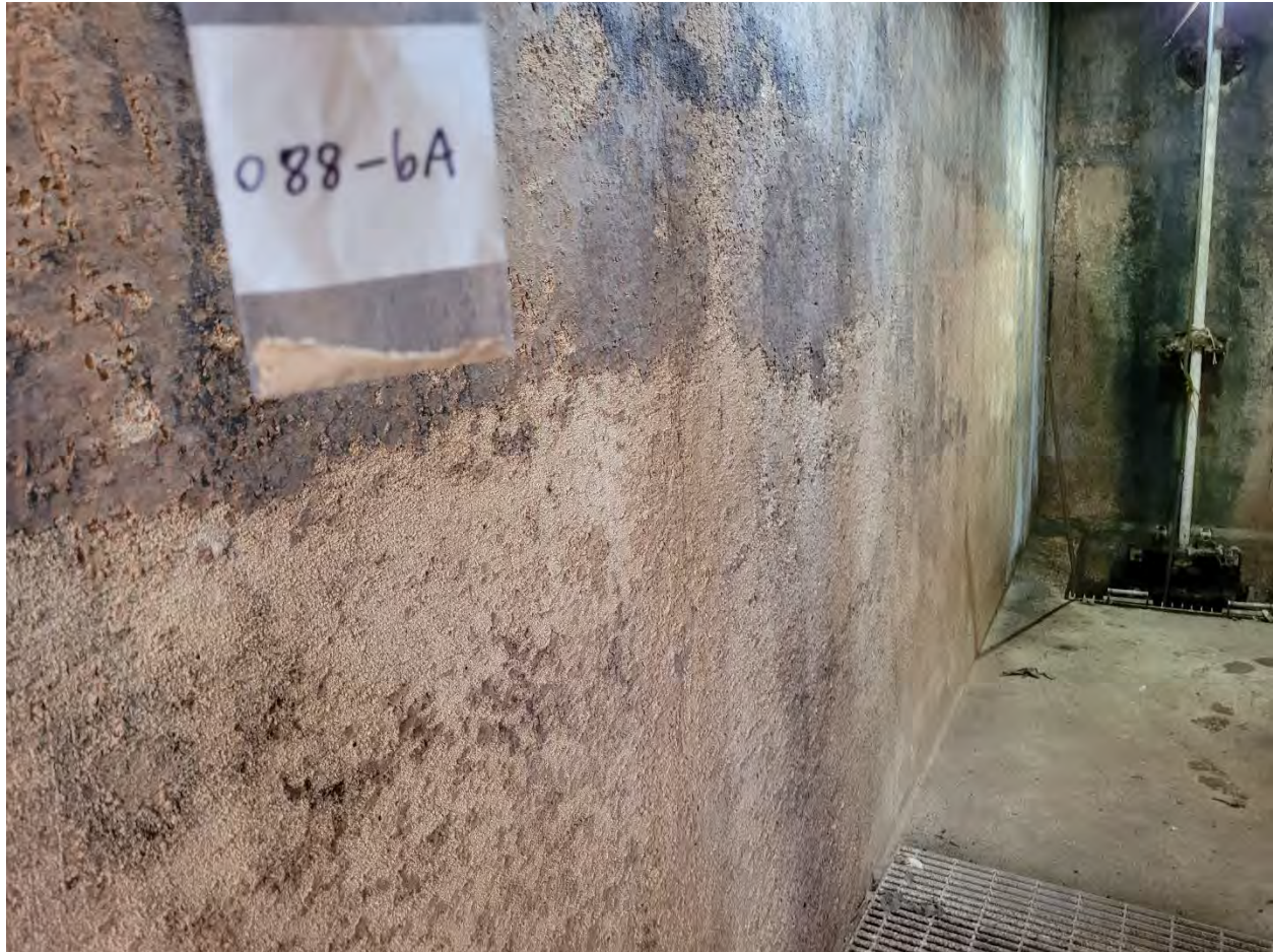
088-6A: Wall Texturing [NAD]
