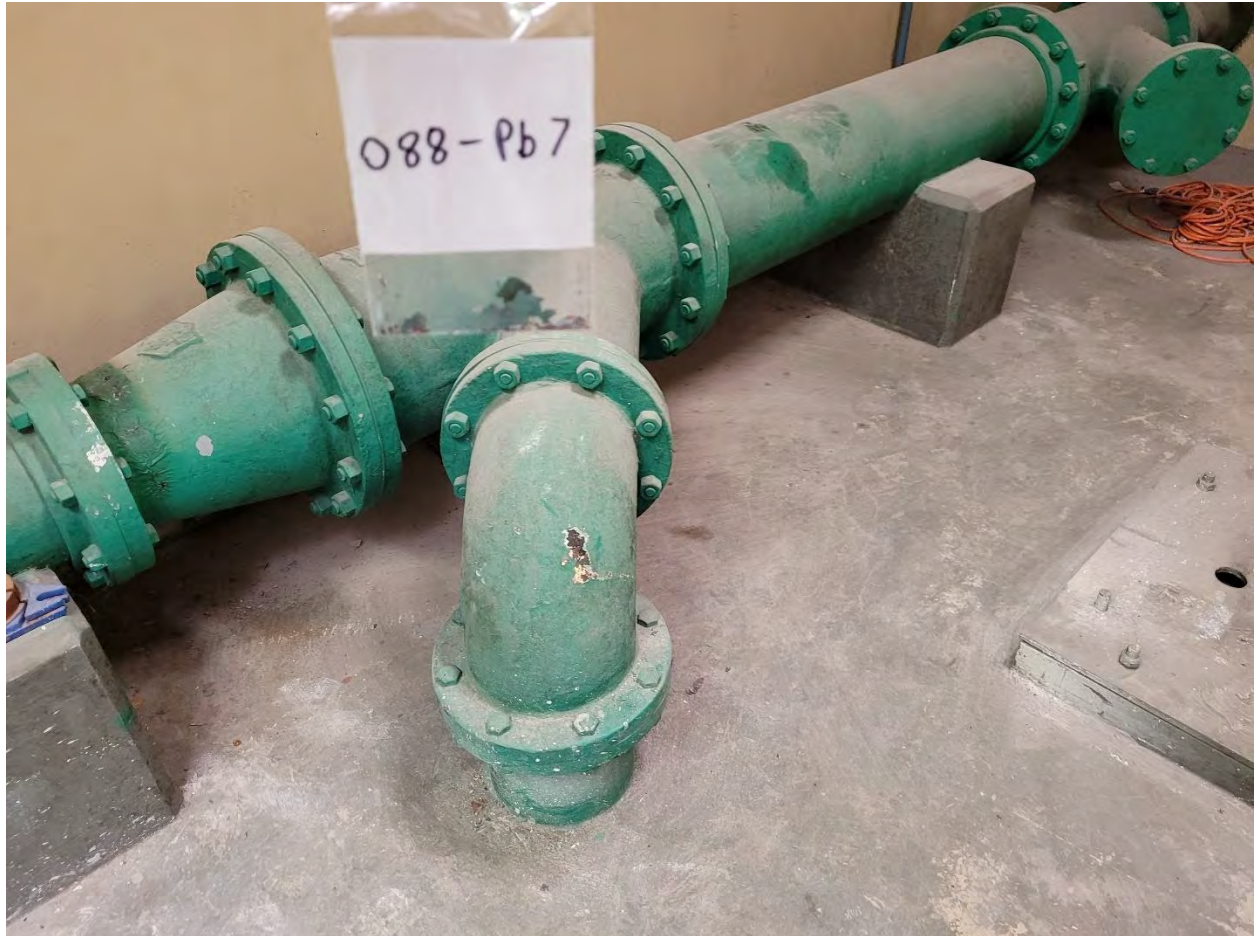
088-PB 7: Green w/ Beige Paint on Metal Pipe [0.064 % wt]
