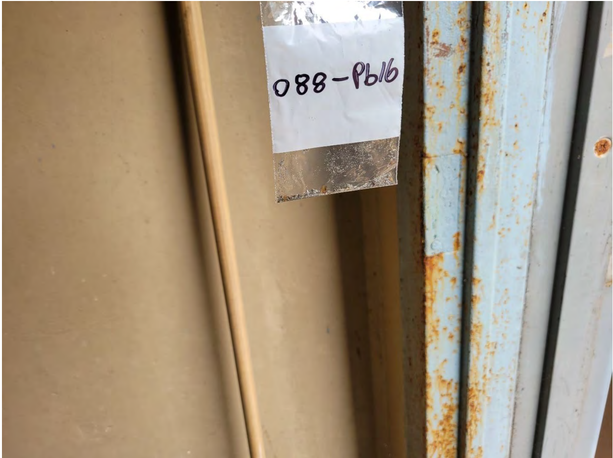
088-PB 16: Light Grey Paint on Metal Frame [0.024 % wt]
