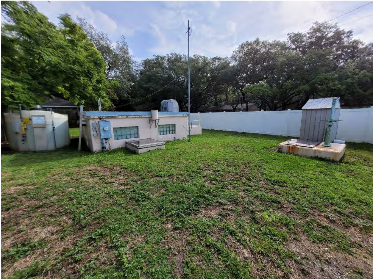
Pump Stat 183: Exterior
