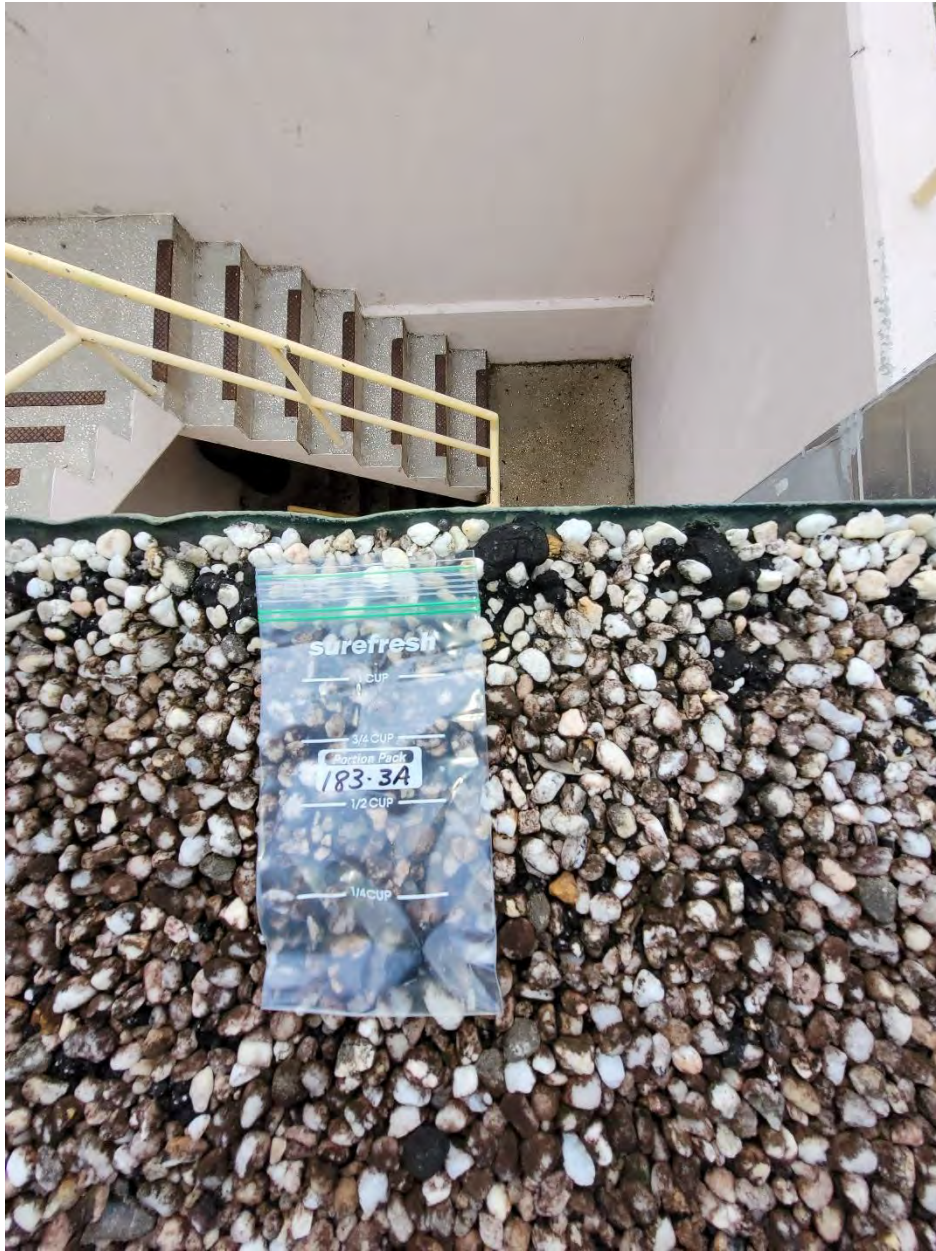
183-3A: Roof Tar [NAD]
