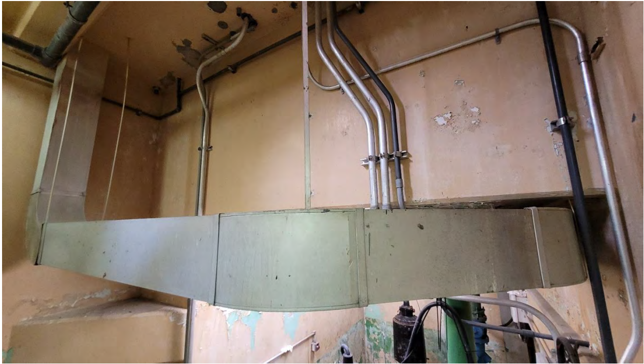
Ductwork should be sampled after the site is inactive
