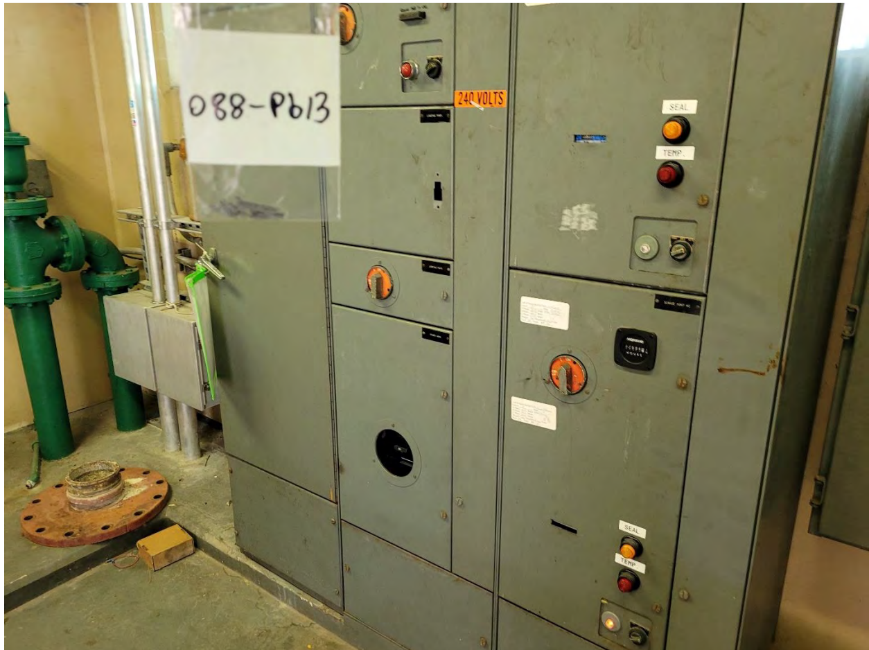
088-PB 13: Grey Paint on Metal Electrical Cabinet [0.21 % wt]
