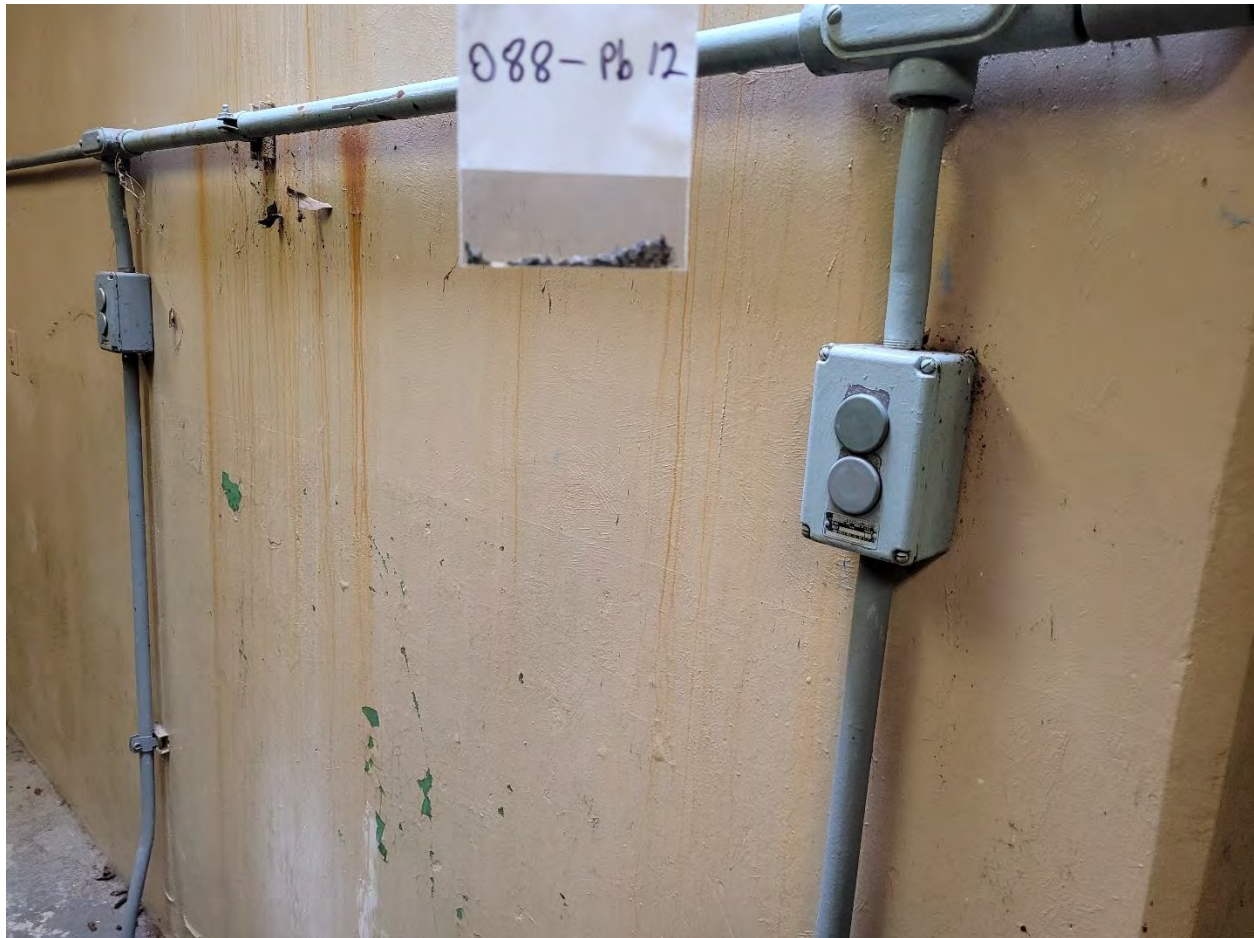
088-PB 12: Grey Paint on Metal Pipe [1.5 % wt]
