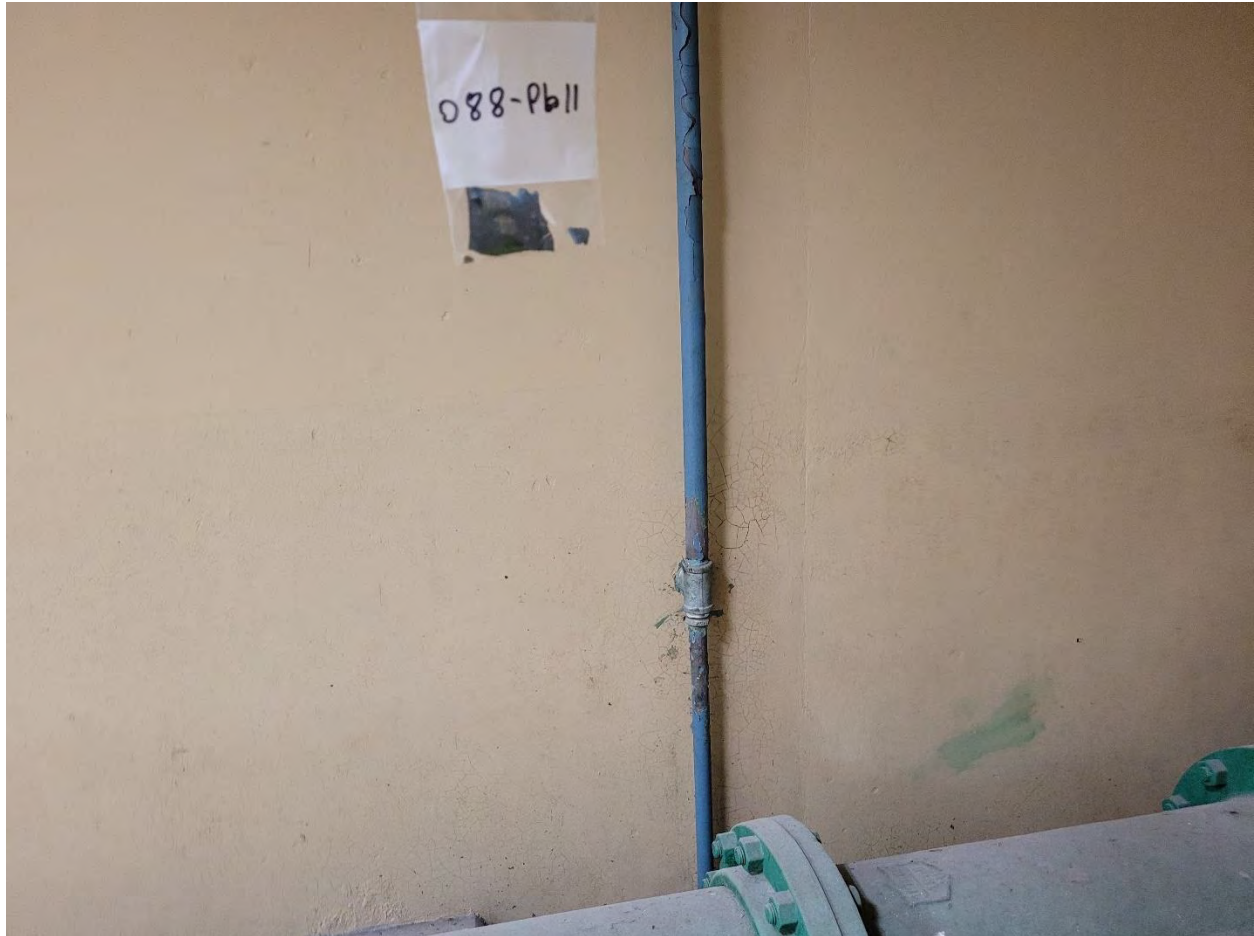
088-PB 11: Blue w/ Green Paint on Metal Pipe [2.2 % wt]
