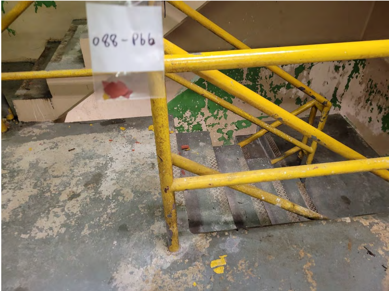
088-PB 6: Yellow w/ Red Paint on Metal Rails [2.4 % wt]
