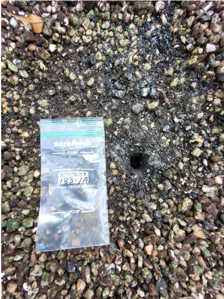
183-1A: Built-up Roof Material [NAD]
