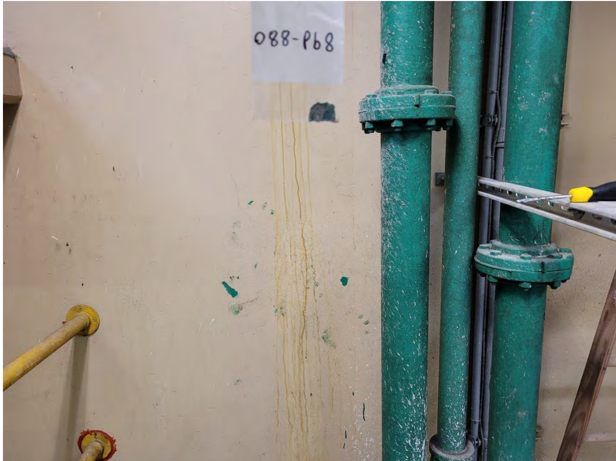
088-PB 8: Green Paint on Metal Pipe [0.028 % wt]
