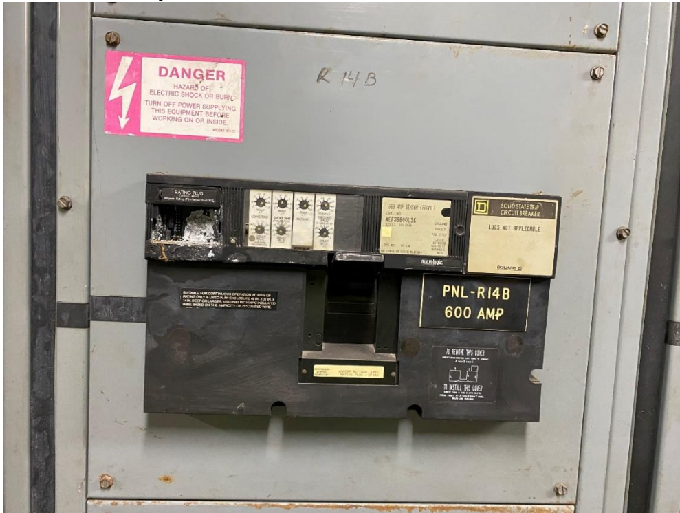
View of (2) MOCP with corroded rating plugs caused by non-conditioned space.
