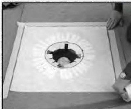
5. Using tape, mask off the termination of the flashing. Catalyzed Parapro Flashing Resin must extend 1/4-inch beyond the Pro Fleece reinforcement, so tape should be placed accordingly. Block the drain opening with paper or tape and cover the bolt holes.
