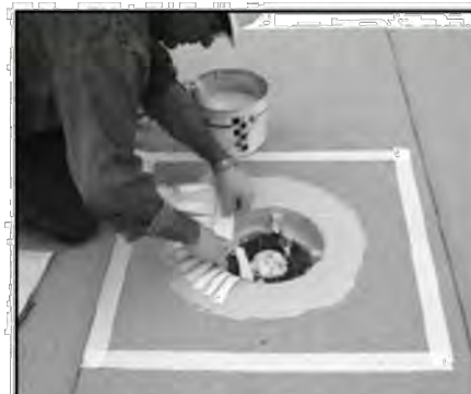
6. Mix the Pro Catalyst and Parapro Flashing as detailed in the mixing instructions. Apply a base coat of catalyzed Parapro Flashing Resin to the prepared drain bowl at a minimum consumption rate of 0.19 kg/sf - 19 kg/sq (0.137 liter/sf), extending onto the roof membrane a minimum of 2 inches. Apply the pre-cut fleece into the drain bowl, ensuring that the resin extends 1/4-inch beyond the edge of the fleece and that no air is trapped beneath the fleece.
