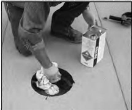
2. Using Pro Prep and a clean shop rag, wipe the area of the drain bowl to be flashed, allow the Pro Prep a minimum of 20 minutes drying time after application before continuing.
