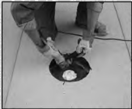
1. Following application of the roof system finish ply, remove all foreign materials from the drain bowl, such as dirt, rust, asphalt, coating, paint or other substances, by grinding. Refer to the substrate preparation chart on page 4 for more information.
