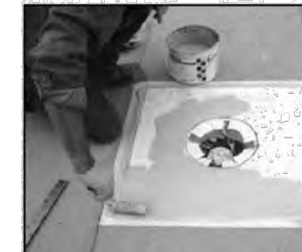
8. Apply the pre-cut Pro Fleece target to the horizontal surface by embedding the fleece in the resin, overlapping the previously applied fleece by a minimum of 2 inches. Ensure that the resin extends 1/4-inch beyond the edge of the fleece, and that no air is trapped beneath the fleece.
