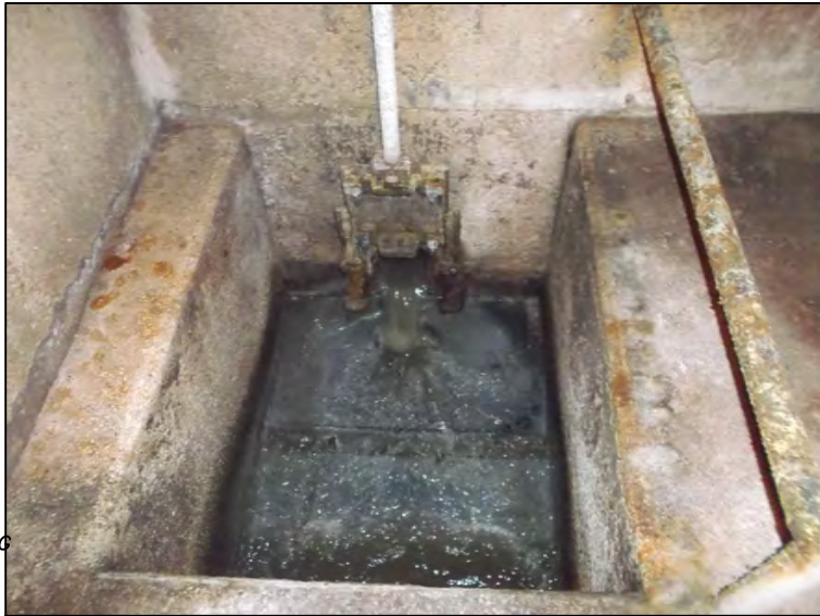
PHOTO OF EX. SLUDGE GATE N.T.S.
