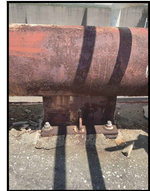
EXISTING PIPE ANCHOR
