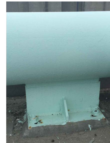
EXISTING PIPE ANCHOR
