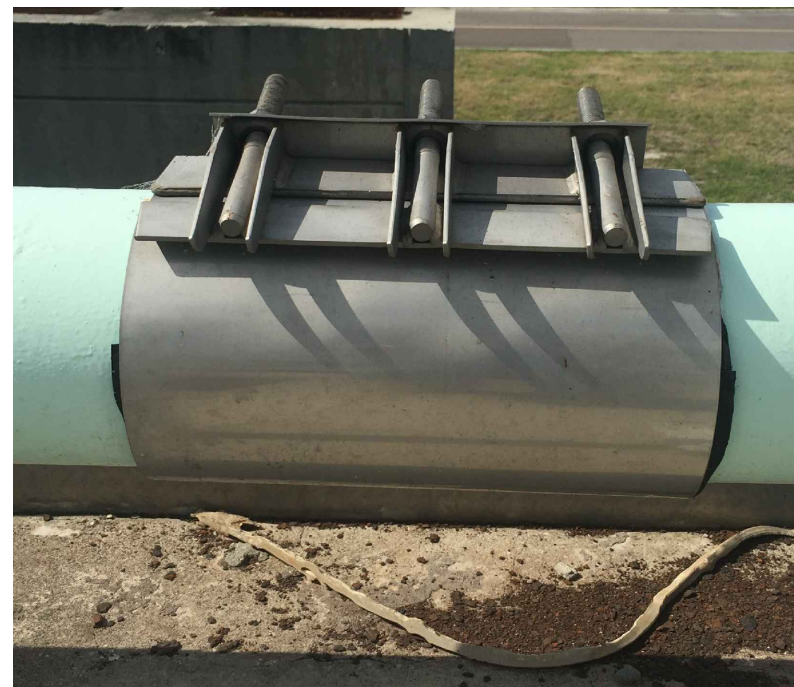
EXISTING STAINLESS STEEL PIPE REPAIR CLAMP N.T.S.
