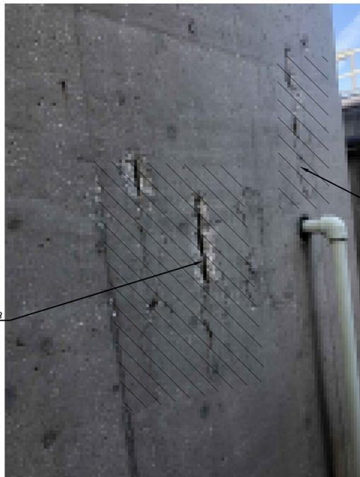
III CONCRETE REPAIR WITH EXPOSED REBAR S-04
