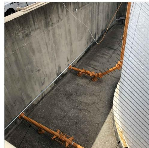
DEMOLISH PIPING WITHIN CONTAINMENT AREA
