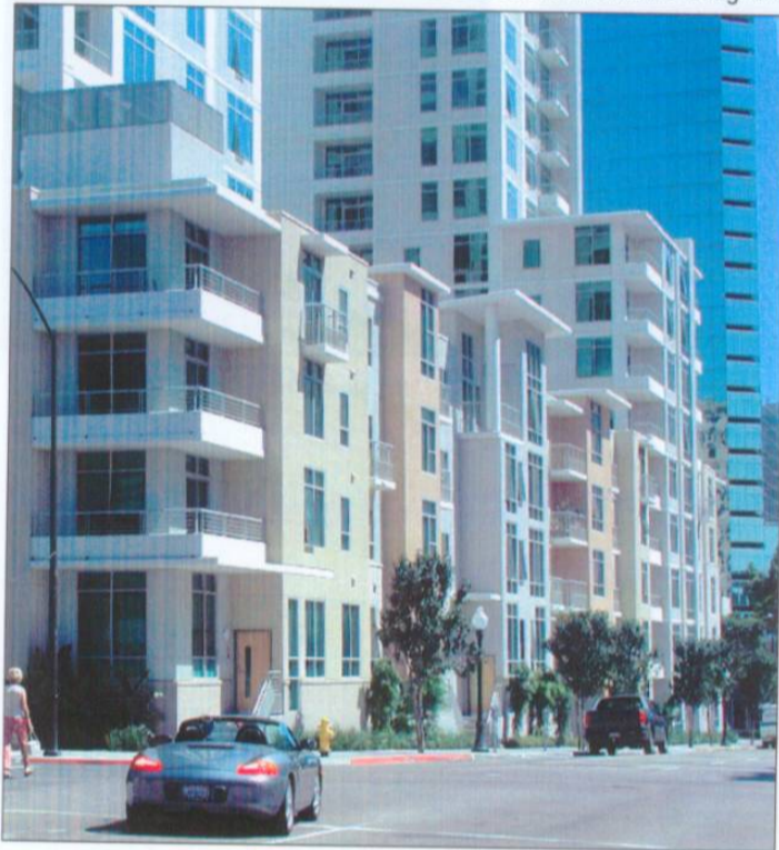
Illustrative Photo: Tower with stoop frontages
