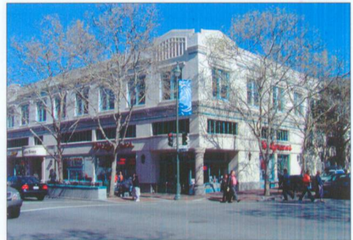
Illustrative Photo: Commercial Block with shopfront frontage
