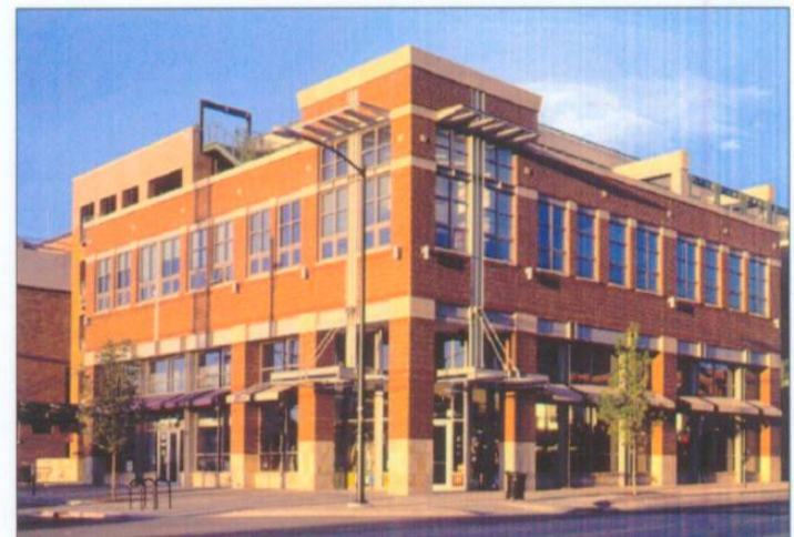
Illustrative Photo: Liner with shopfront frontage
