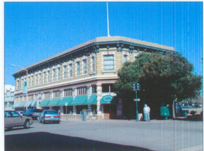
Illustrative Photo: Commercial Block with shopfront frontage
