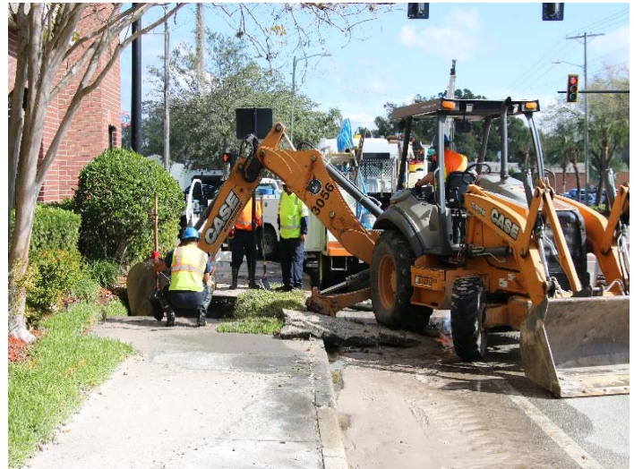
Water Main Break Repair
