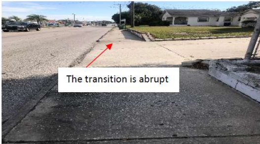
Driveway Apron Reconstruction
