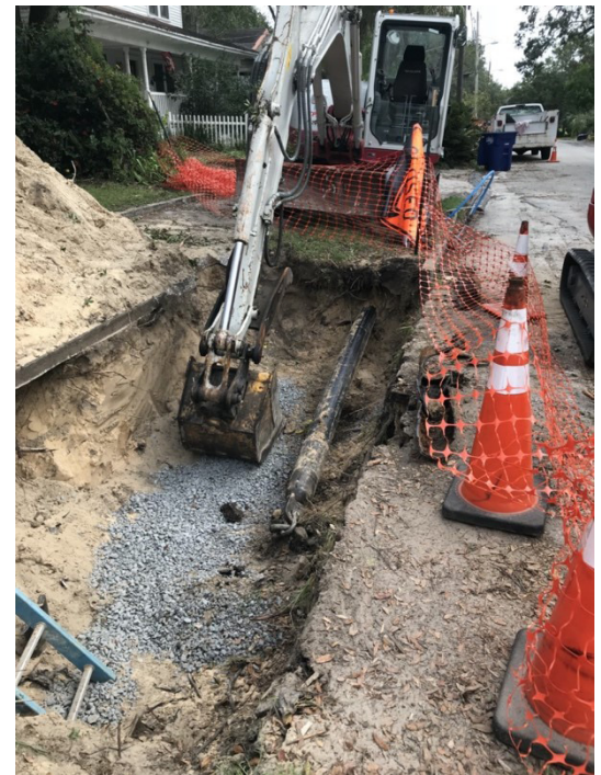
Repair work on Water Pipes
