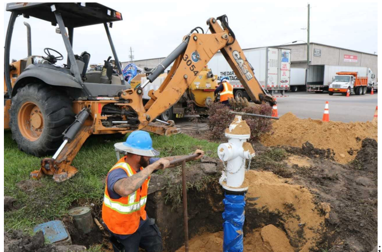
Water Hydrant Installation
