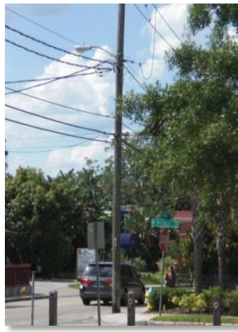
Figure 2-23 Cobra Head Lights
