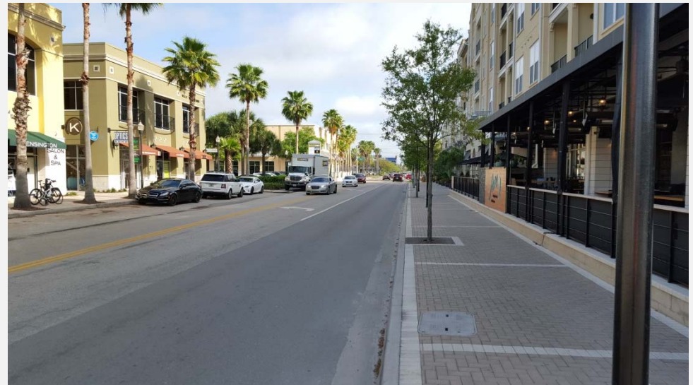
South Howard Avenue between W. Morrison Ave. and W. Swann Ave.
