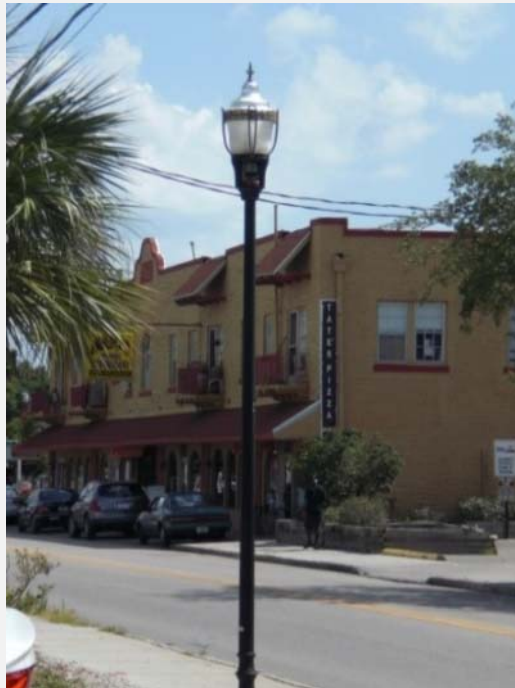
Post Top Ornamental Lights
