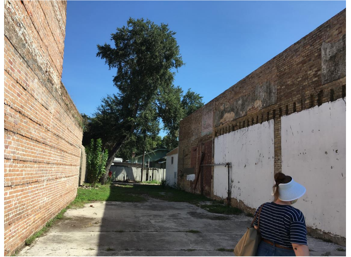
This street has some unused open spaces between the shops.
