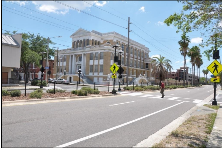
Figure 10-1 - E Palm Avenue and N 17th Street – Pedestrian using RRFB at mid-block crosswalk
