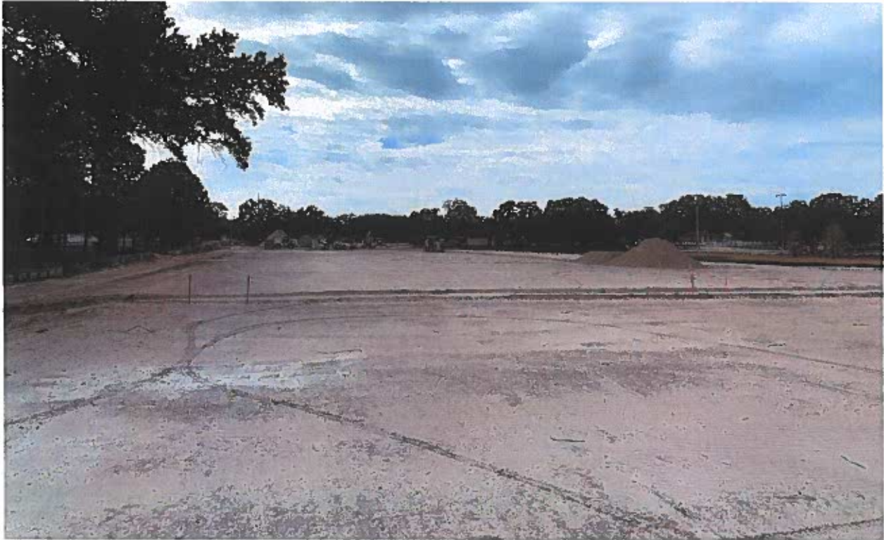
Fine Grading at Multipurpose Field
