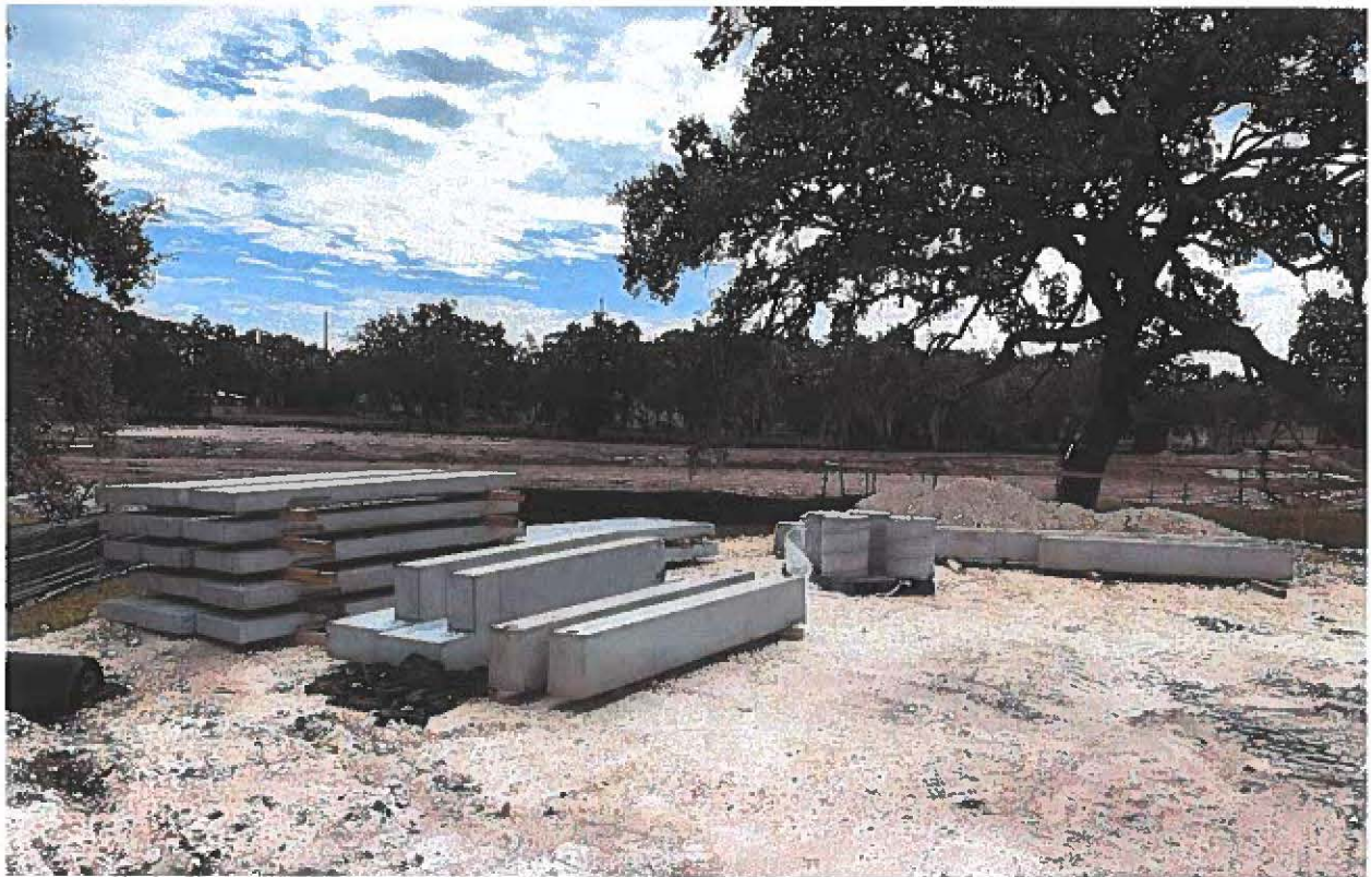
Pedestrian Bridge Precast Concrete Pieces on Site
