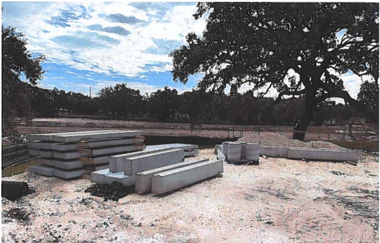
Pedestrian Bridge Precast Concrete Pieces on Site
