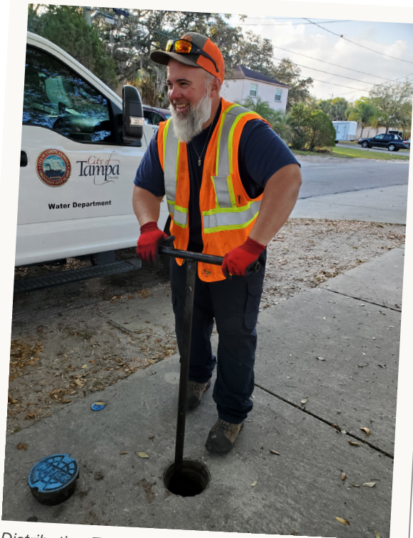
Distribution Technician opening a water valve
