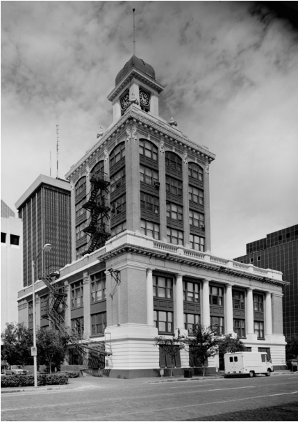
The 1982 renovation of City Hall removed the fire escape and Bahama shutters, which were added to the building in 1962.
