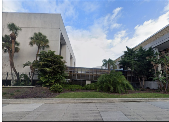
Tunnel connecting annex and library (Google Maps 2019)
