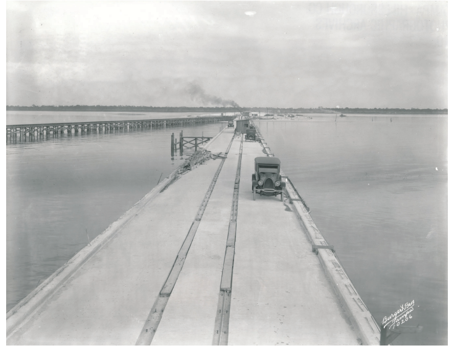
Gandy Bridge under construction over Old Tampa Bay on December 17, 1923.
