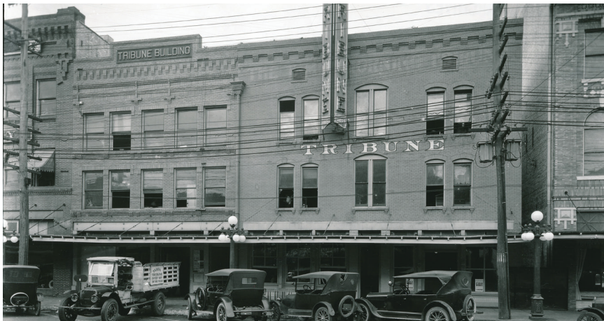
Tribune Building on Tampa Street (500 block), three story brick front façade, March 15, 1923.
