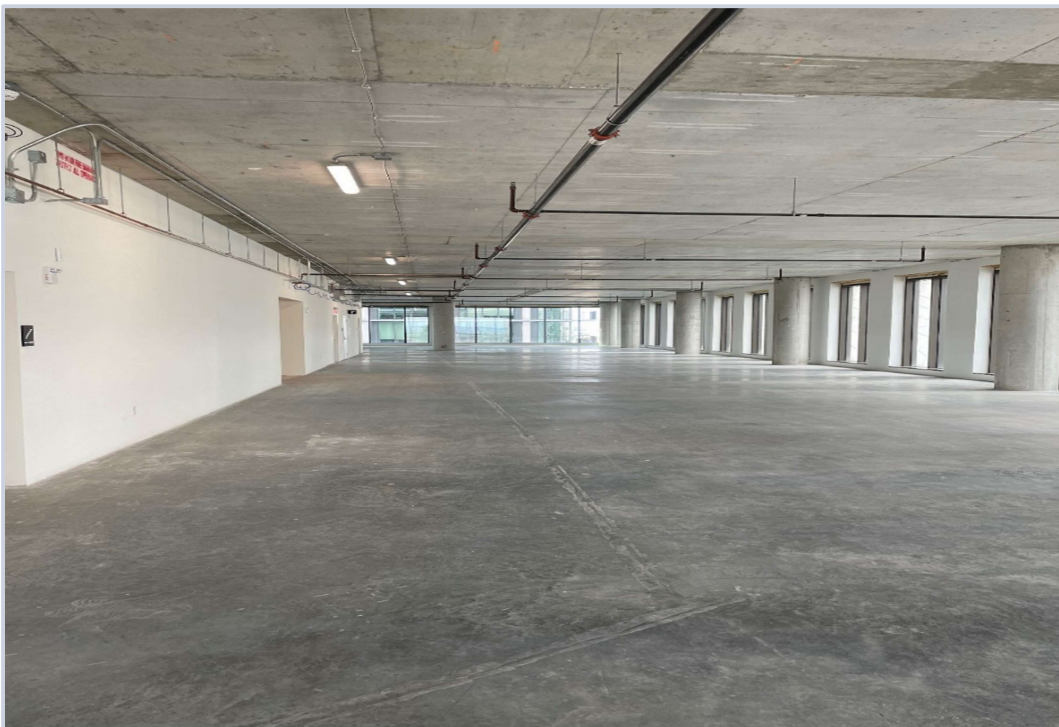
Example of a Shell Building
