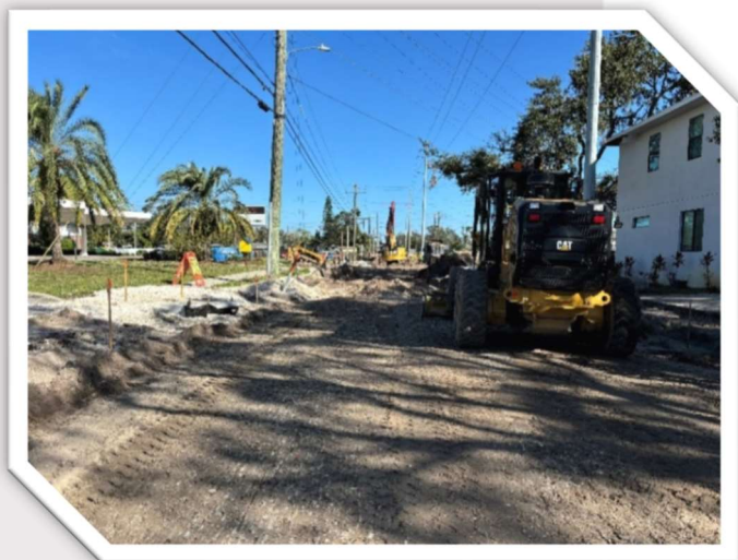
Himes Ave – Box and Culvert Installation
