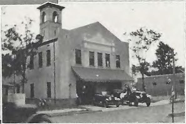
Florida Avenue Station No. 5
