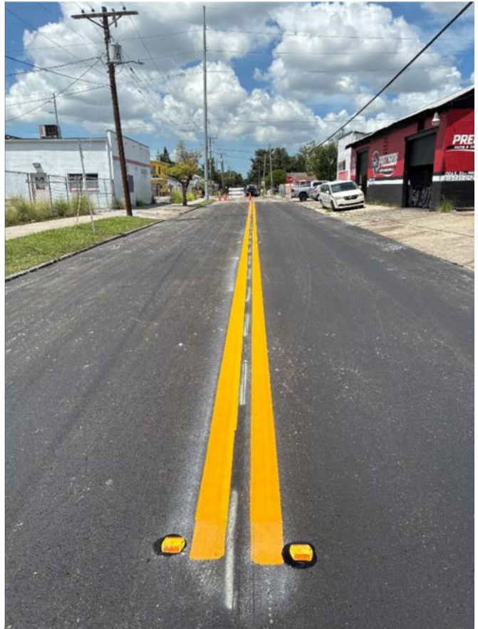
Utility Cut Out Paving - Stormwater Cave-In - 710 W. West St.
