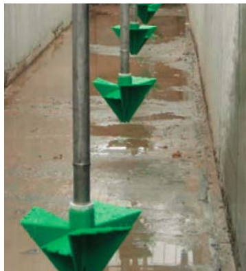
Figure 5.1-7: Photo of EDI HexAir Coarse Bubble Diffusers
