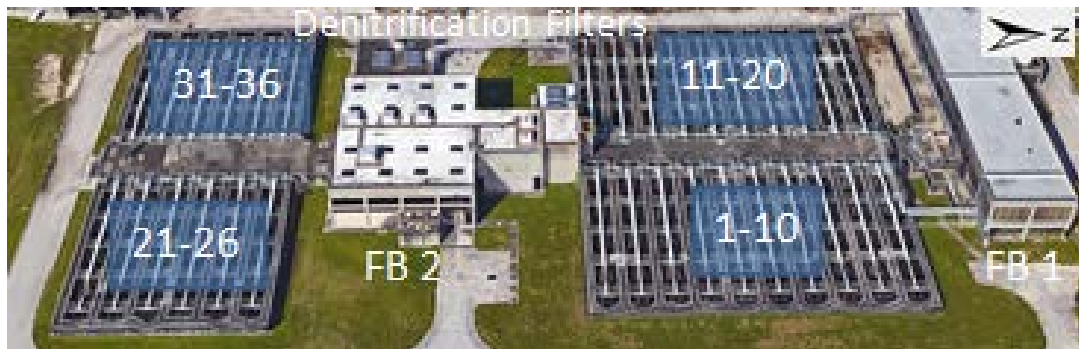
Figure 8.1-1: Existing Denitrification Filters
