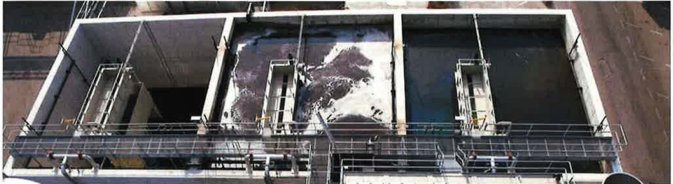
Figure:1 Modular AnammoPAQ™ setup at Rendac, The Netherlands (13,000 lbs N/day)
