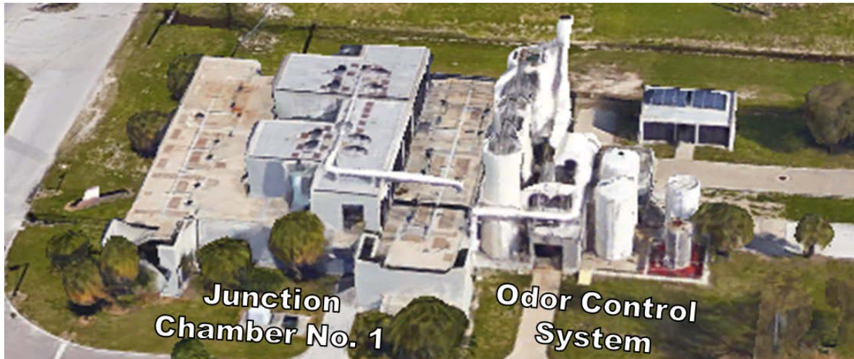
Figure 5.1-1: Junction Chamber No. 1
