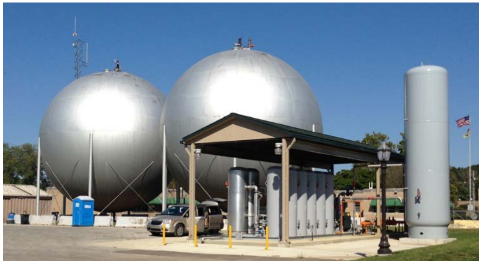
Figure 12.4-7: Example Microgate PSA RNG System (75 SCFM)
