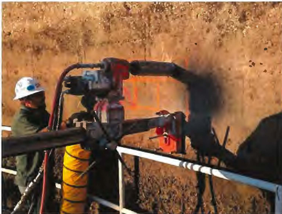
Photo 4 – Hydraulic core machine mounted on the wall.
