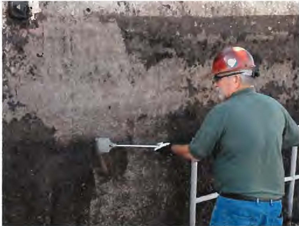
Photo 3 – Scraping the walls prior to half-cell testing.
