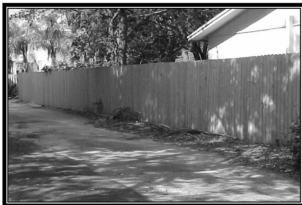
Unpainted Wood Fencing is inappropriate.
