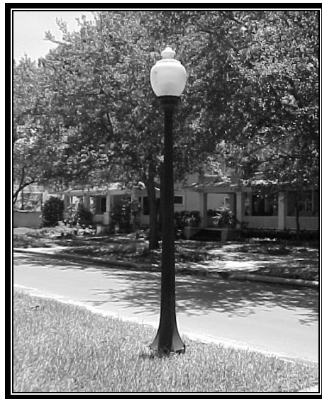
Typical Style Street Light
