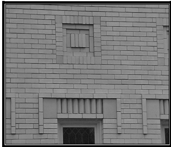
Typical Brickwork Detail
