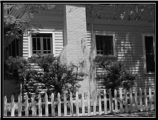
Window Placement which adds to the interior & exterior appearance of the house.
