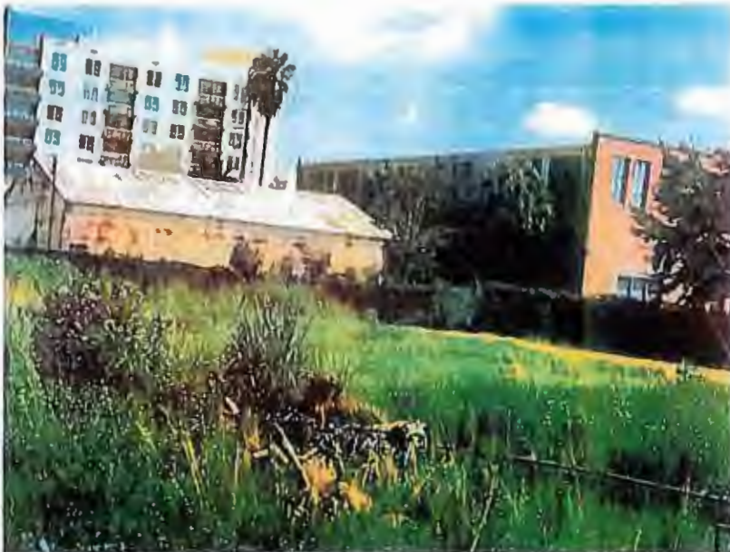
(Both deteriorating parcels shown in picture below)
