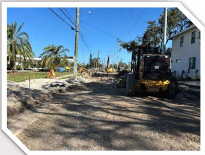
Himes Ave – Box and Culvert Installation
