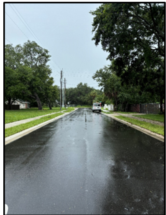
Averill Road – Complete Restoration
