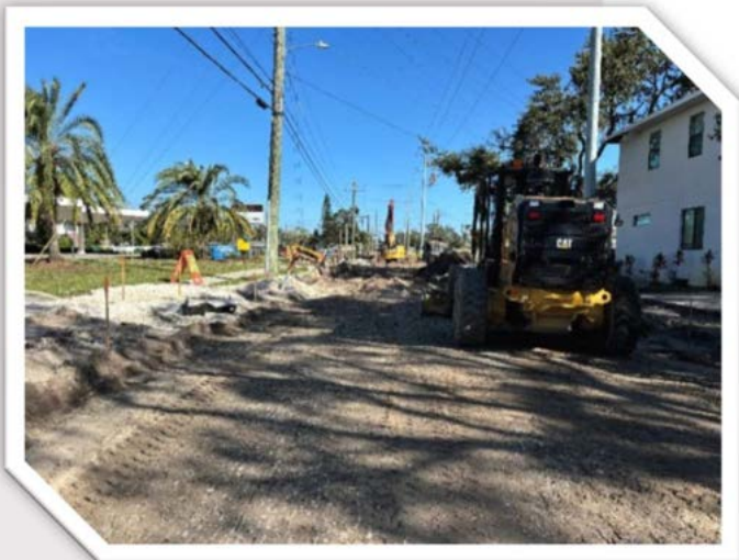
Himes Ave – Box and Culvert Installation
