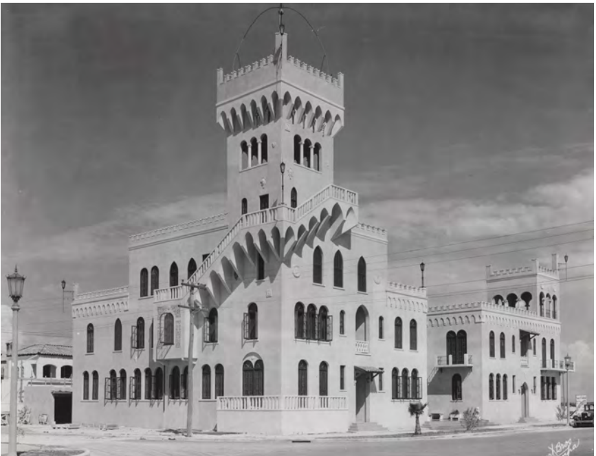
The Palace of Florence Apartment Hotel was completed in 1926 on Davis Islands. This photo shows a side view of the multi-story Mediterranean Revival building, which still stands today.
