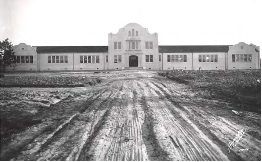
Ballast Point School under construction at 2702 Ballast Point Boulevard on March 3, 1926.
