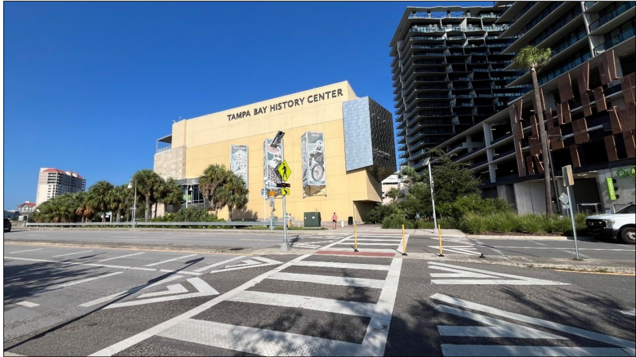
Figure 4-1. Existing At-Grade Crossing along Beneficial Drive
