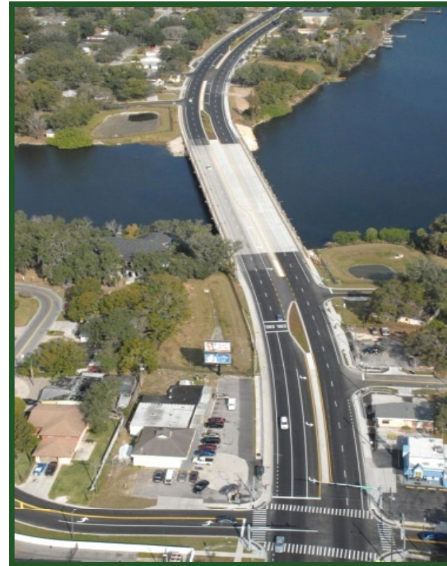
40th Street Segment After Construction
