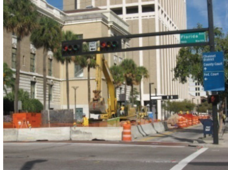
Replacing Aging Water Mains Downtown
