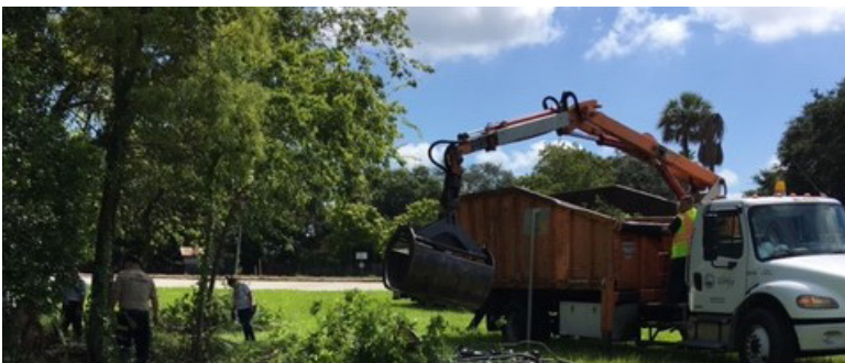
Neighborhood Enhancement Clearing Overgrowth
