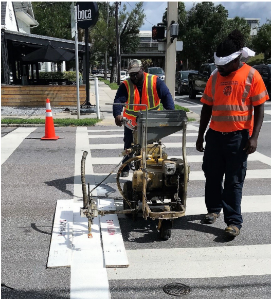
Smart Paint Application at Platt Street
