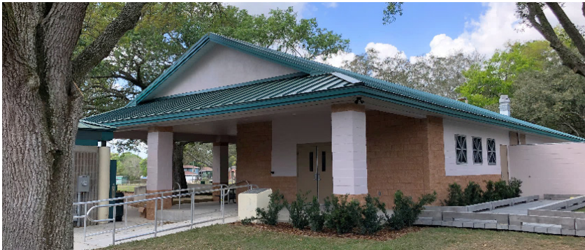
Building Addition at Williams Park
