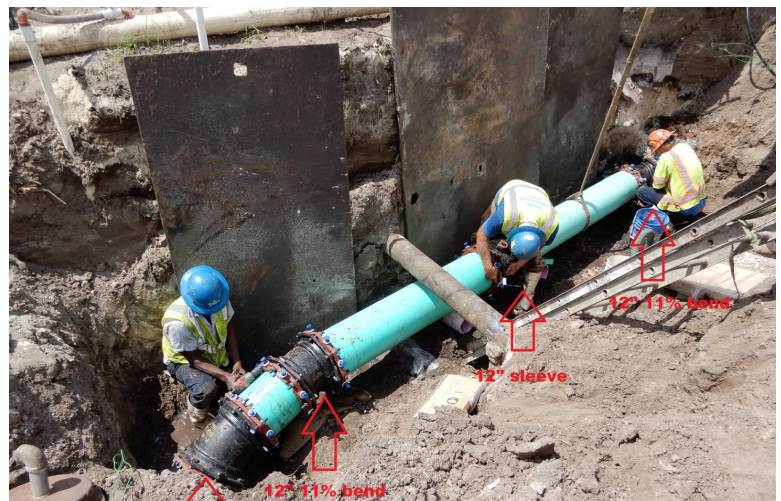
Orient Road Force Main Replacement
