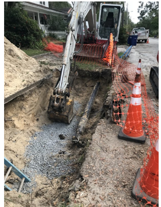
Repair work on Water Pipes
