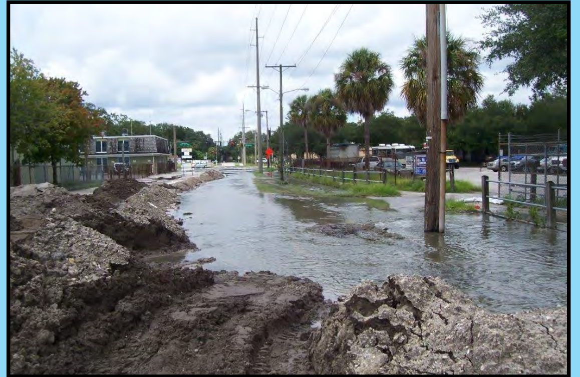
University Pump Station Force Main Break
