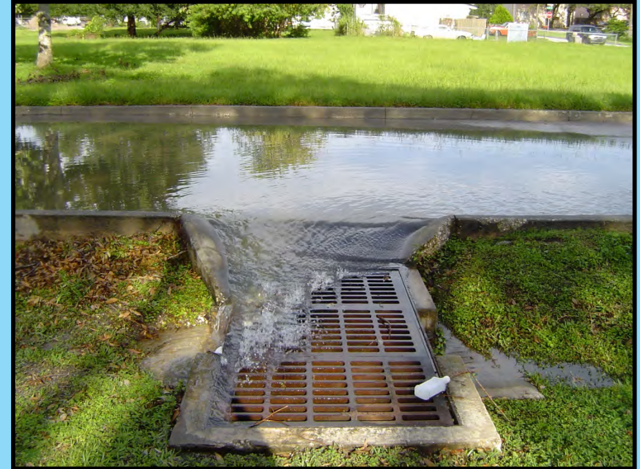
Overflow going directly into the Stormwater System
