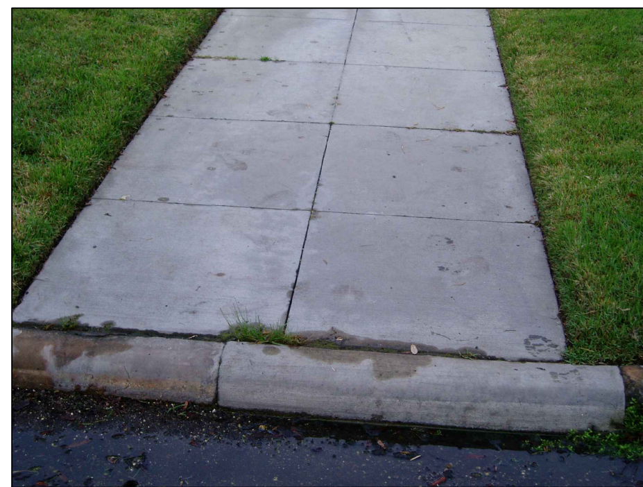
EXAMPLE OF SIDEWALK RECONSTRUCTION
