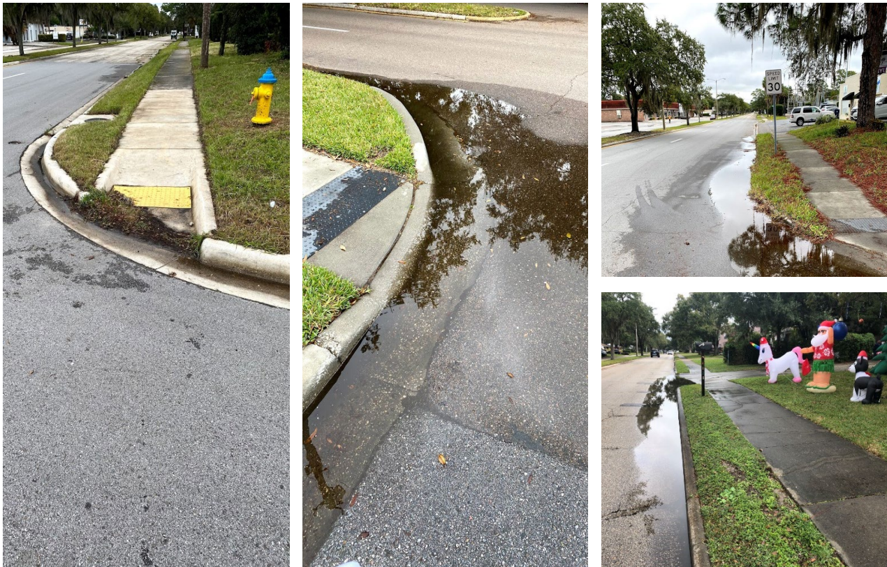
Figure 15: Ponding and sediment in walkways and bikeways create obstacles that reduce the viability of alternate modes
