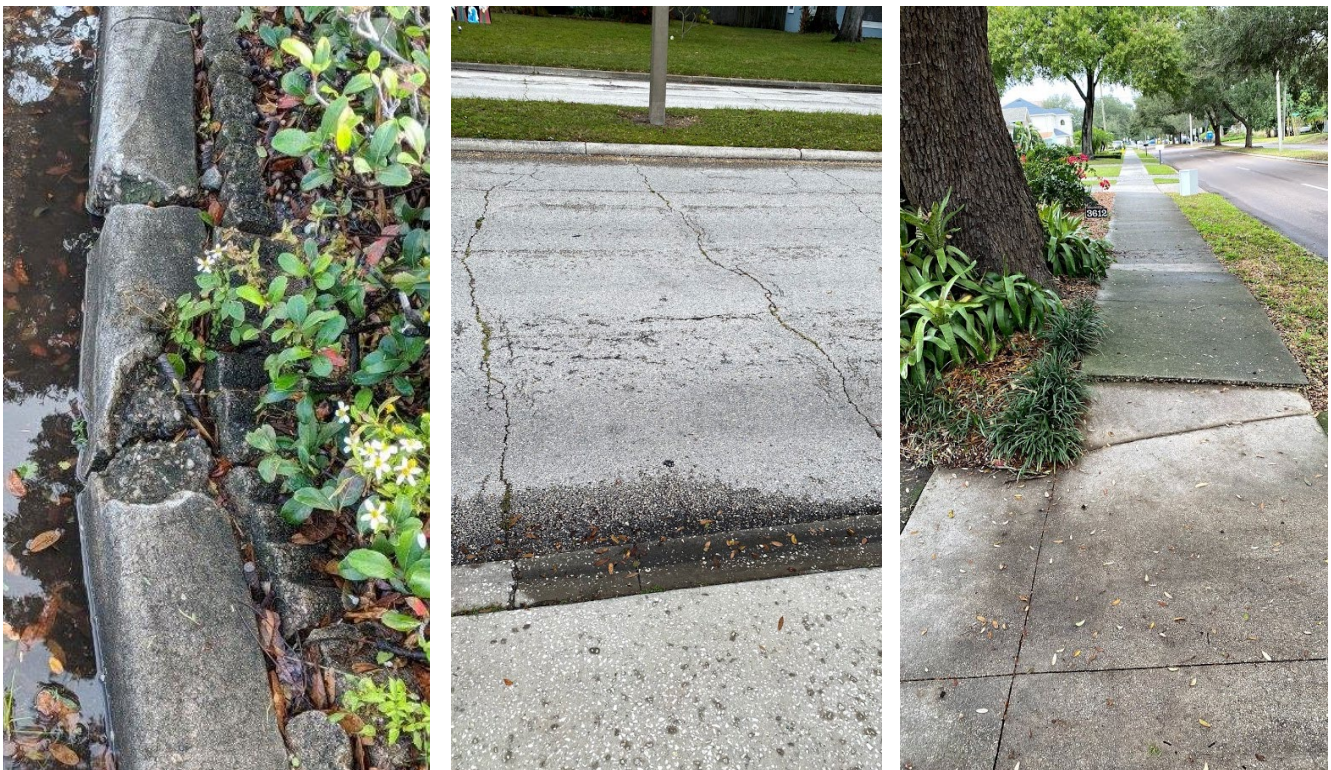
Figure 16: The City will look to rehabilitate the corridor assets; broken curb, pavement failures, and upheaved sidewalks should be evaluated for correction.
