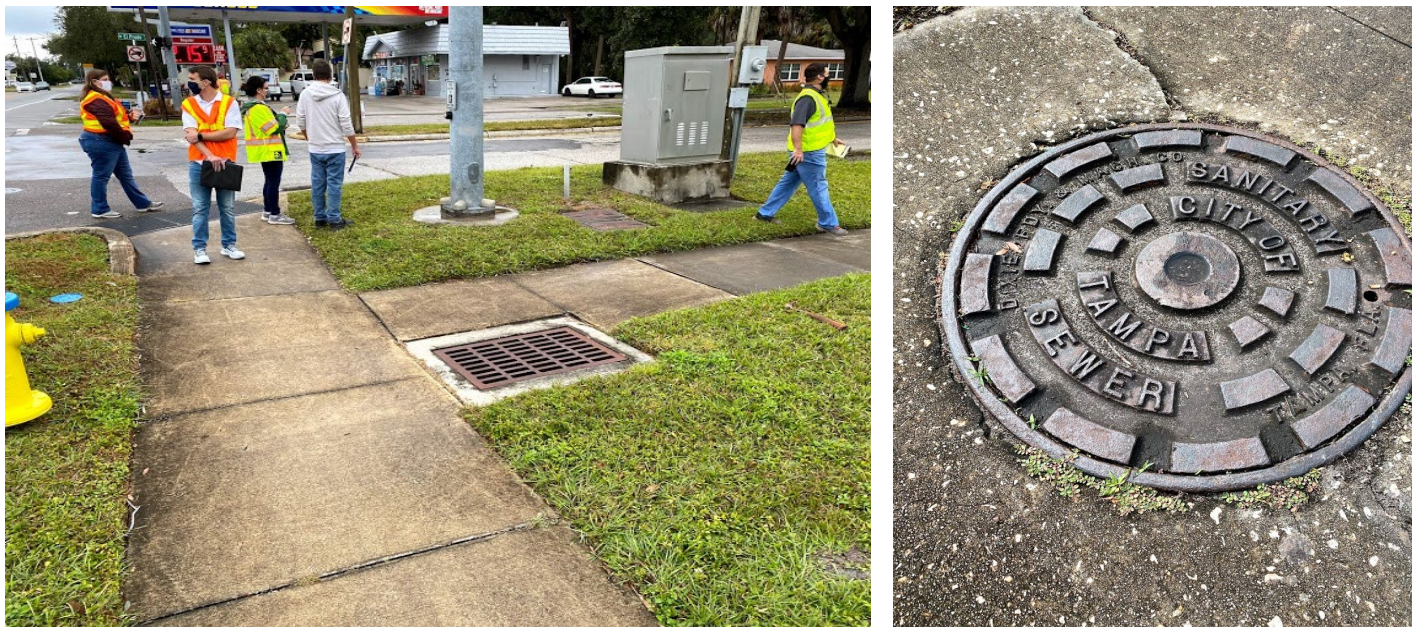
Figure 8: Drainage inlet within sidewalk in area of sidewalk swale (left); sanitary sewer manhole cover within southside sidewalks (right)
