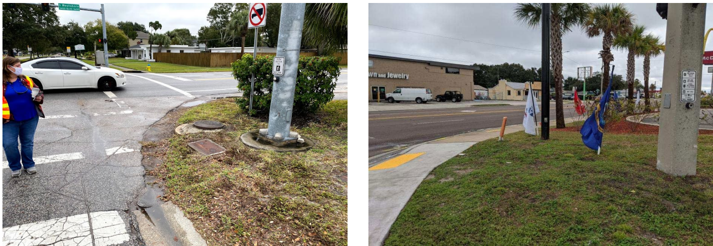
Figure 9: Inaccessible push buttons at West Shore Blvd. and Dale Mabry Hwy, left and right, respectively
