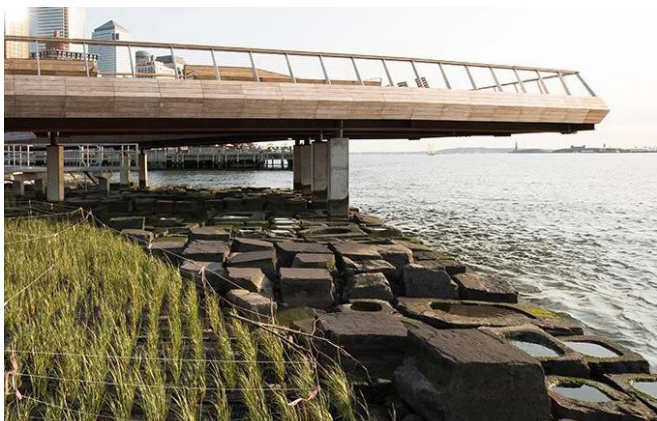
Concrete reef coastline example using EConcrete at Pier 26, New York City, NY
