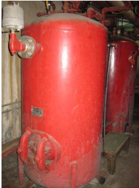
**Figure 4-6: Pressurized Biogas Condensate/Sediment Trap**
