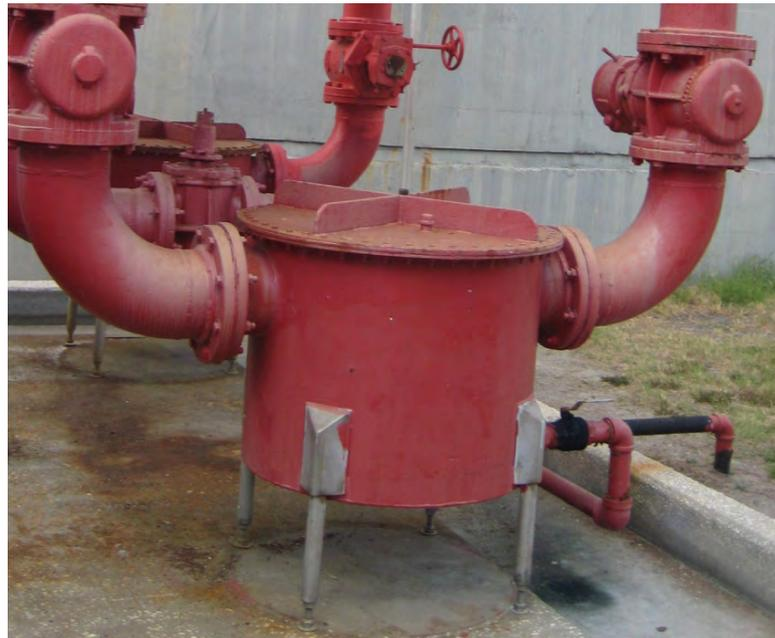
**Figure 4-4: Biogas Condensate/Sediment Trap**
