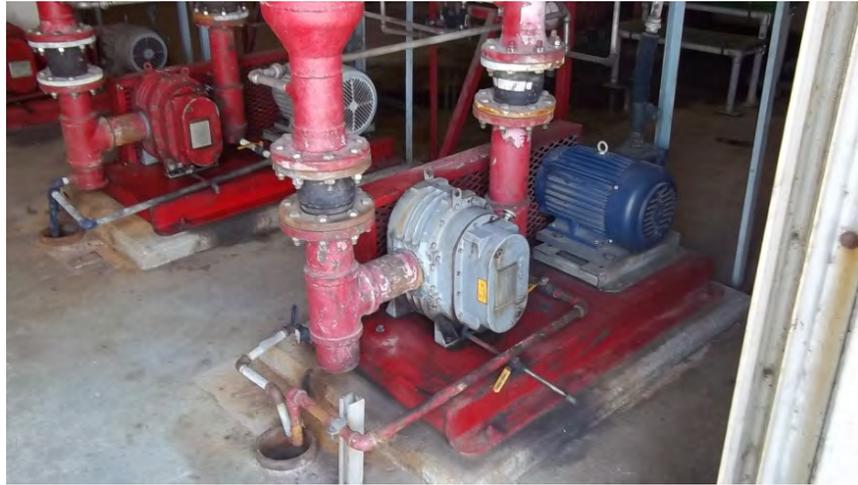
**Figure 4-2: Biogas Compressors**
