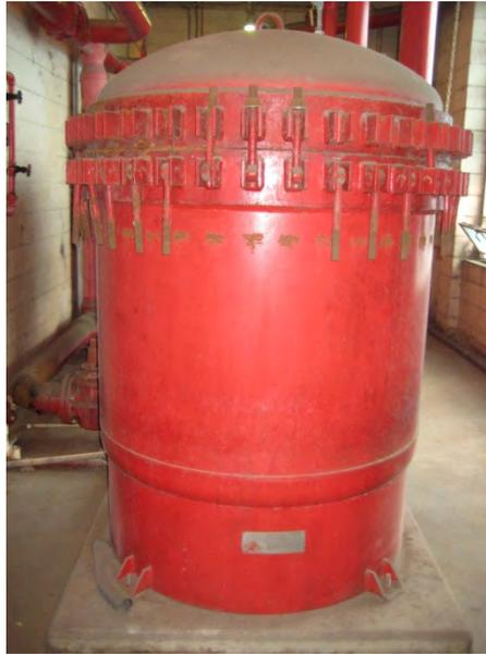
**Figure 4-3 - Biogas Conditioning Filter**
