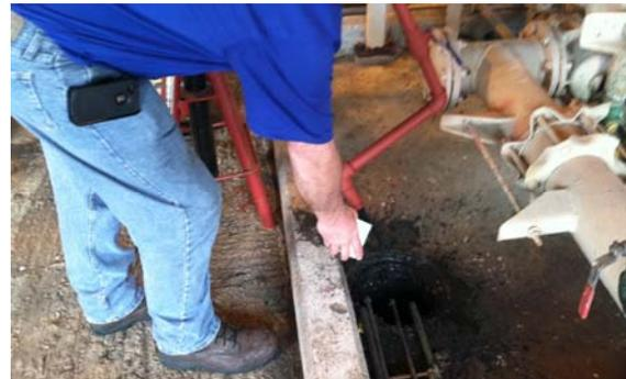
**Photo 2: Feed Sludge Sampling**
