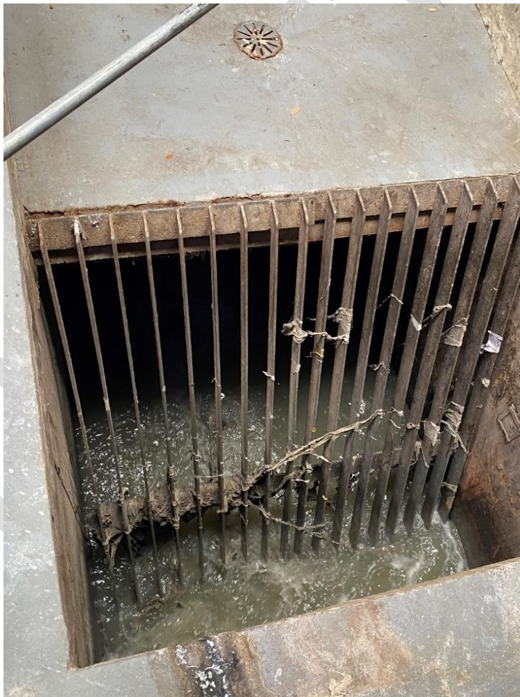
FIGURE 1: EXISTING MANUAL COARSE SCREEN
