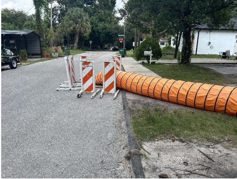
Photo 4-14 Temporary Duct Connection to Influent MH
