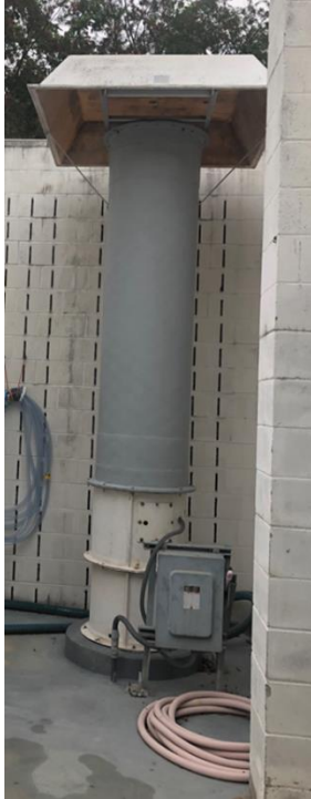
Photo 5-3 SSPS Wet Well Intake Vent
