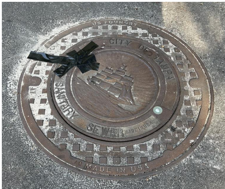
Photo 5-1 Manhole With Differential Pressure Monitor Installed
