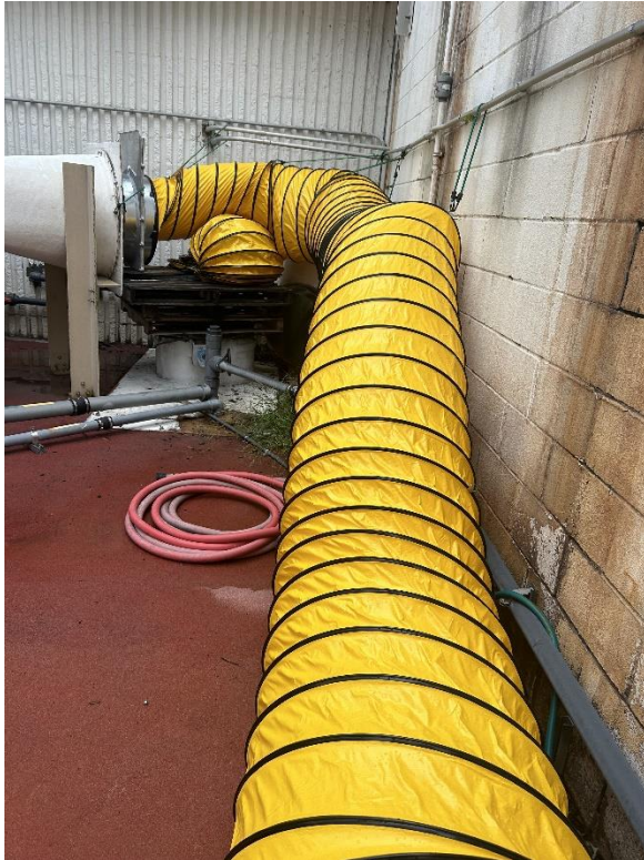
Photo 4-12 Temporary Duct Connection to OCF
