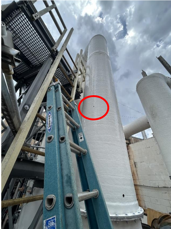
Photo 4-10 SSPS Air Flow Sampling Location
