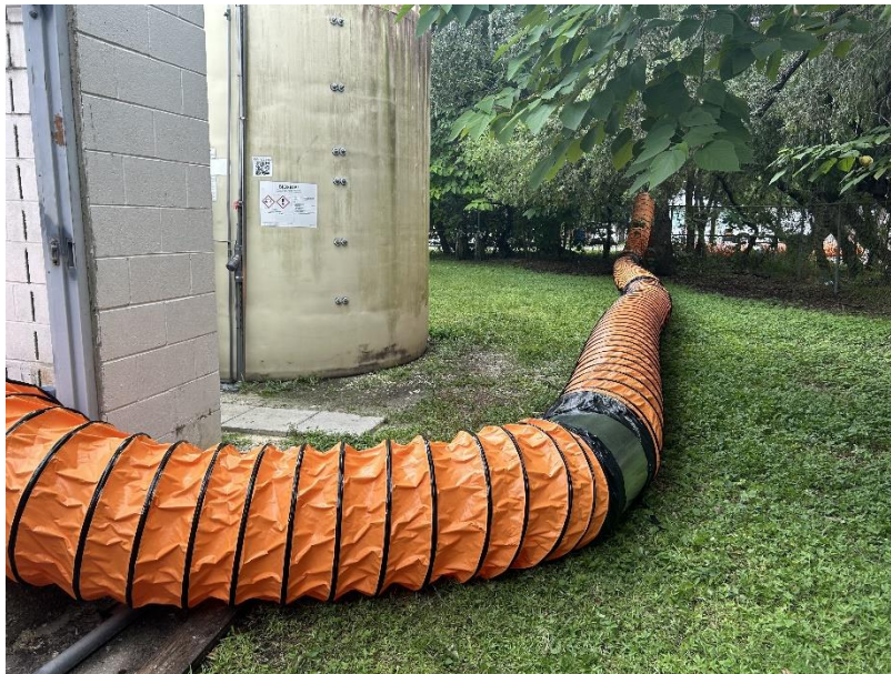
Photo 4-13 Temporary Duct Routing to Influent MH
