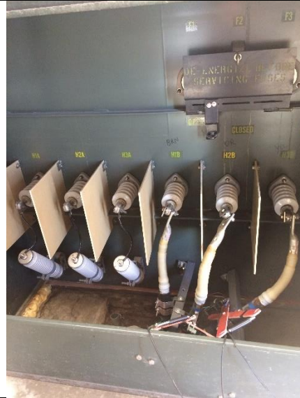
Photo of Sensor Attachment
