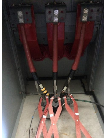
Photo of Sensor Attachment
