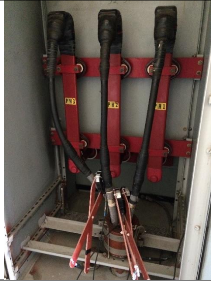
Photo of Sensor Attachment
