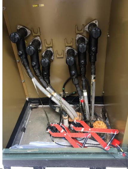
Photo of Sensor Attachment
