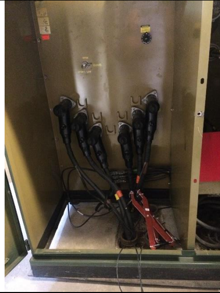
Photo of Sensor Attachment
