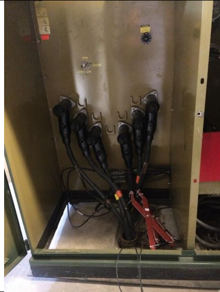
Photo of Sensor Attachment
