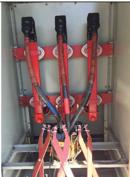
Photo of Sensor Attachment
