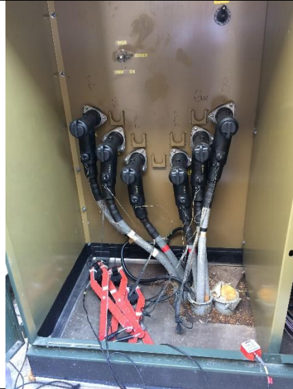
Photo of Sensor Attachment
