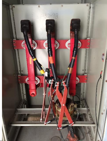
Photo of Sensor Attachment
