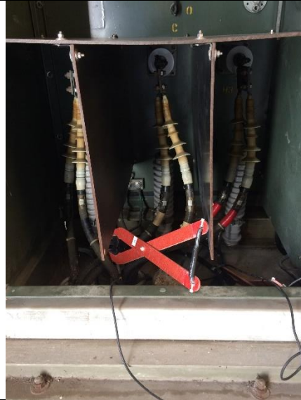
Photo of Sensor Attachment
