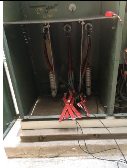
Photo of Sensor Attachment
