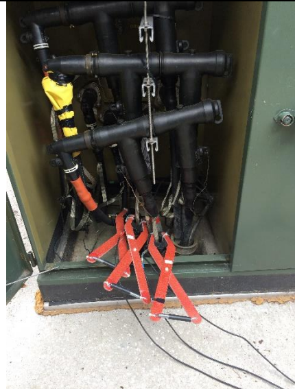
Photo of Sensor Attachment
