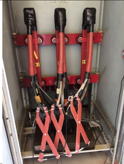
Photo of Sensor Attachment
