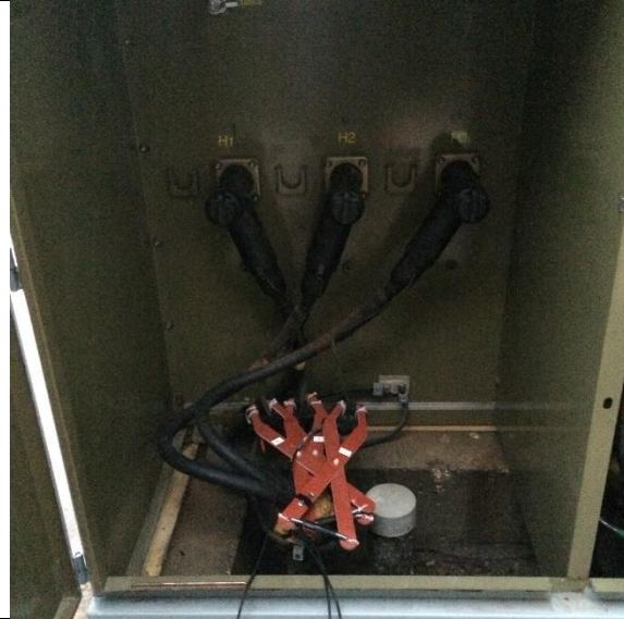
Photo of Sensor Attachment
