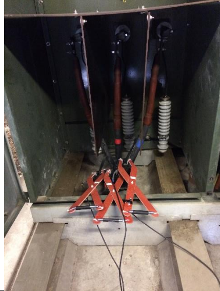
Photo of Sensor Attachment
