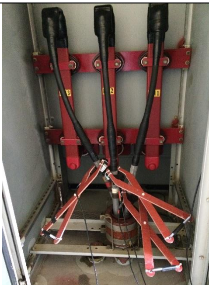
Photo of Sensor Attachment
